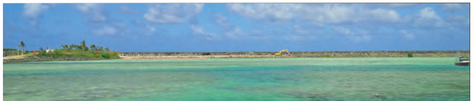
A view of the Agana Small Boat Harbor breakwater repair that was a topic of discussion between District leadership and Guam government officials during visits in September and October. Courtesy photo
