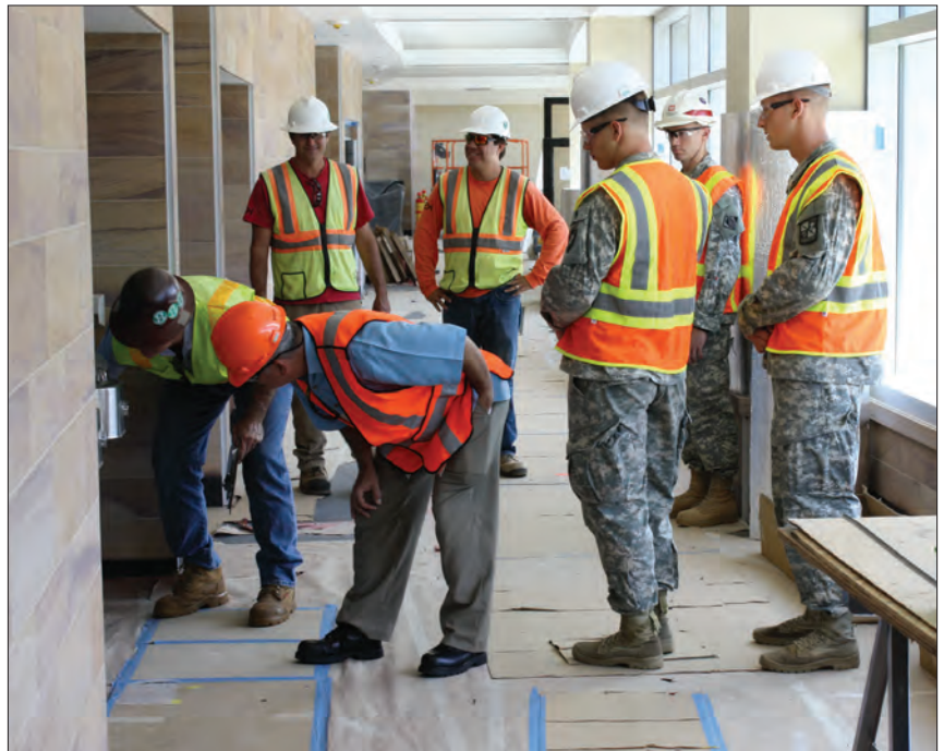
Cadet Walker Glunz (right) and Cadet Calvin Kiesewetter (third from right) observe contractors inspecting a water fountain drain line inside the USARPAC Mission Command Facility (MCF) project at Fort Shafter. Photo by Dino W. Buchanan
