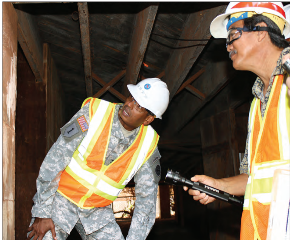
Honolulu District Supervisory Engineer Steve Yamamoto shows U.S. Army Pacific Commander Gen. Vincent K. Brooks World War II graffiti painted on a pillar in the basement Fort Shafter's Bldg. T-112 . Building T-112, built in 1907 and also known as Dunning Hall, is an important structure in the Palm Circle National Historic Landmark District. Photo by Joseph Bonfiglio
