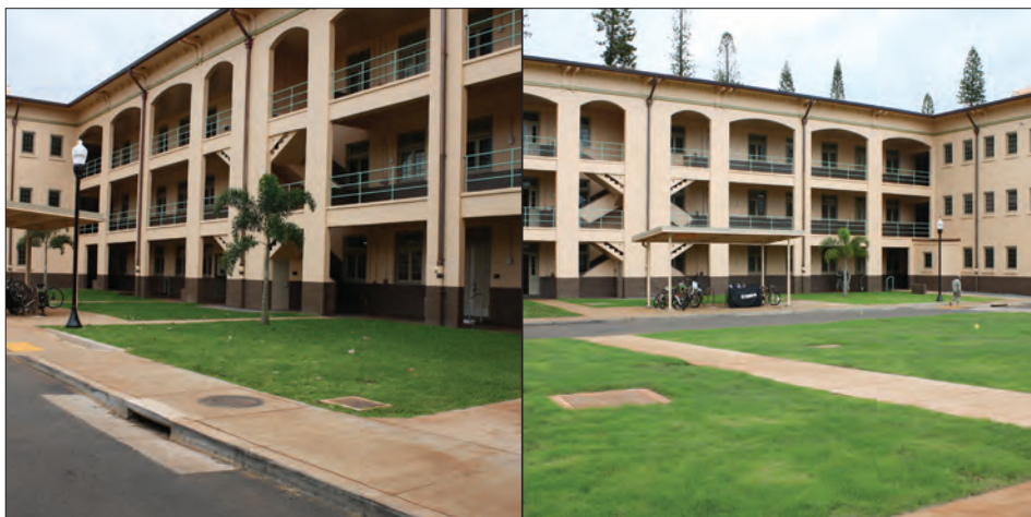
The rehabilitation of Buildings 450 (left) and 451 (right) of Quad D are part of U.S. Army Garrison Hawaii's Whole Barracks Renewal Program, which aims to restore the five historic barracks on post, including one (Quad B) that was built in 1914. Photos by Dino W. Buchanan
