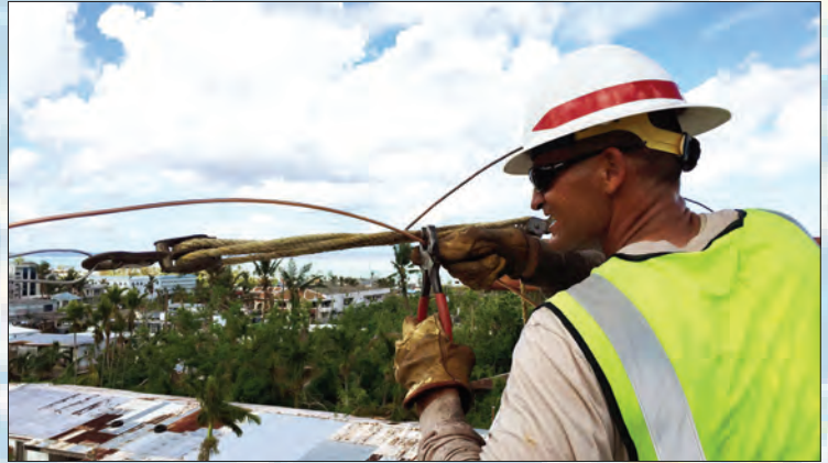
Delta Company's Cpl. David Schmidt repairs an electric line that powers water wells in the Gualo Rai area of Saipan. Courtesy photo
