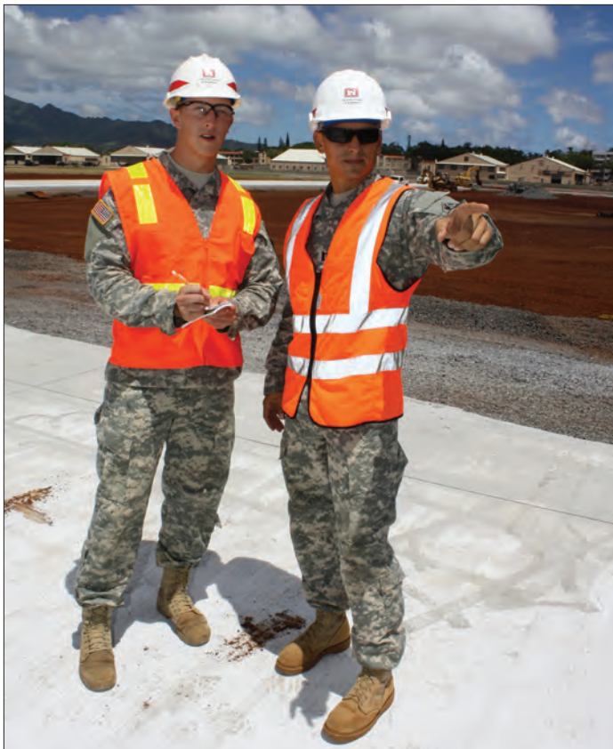
Cadet Walker Glunz (left) takes notes about the Combat Aviation Brigade Phase 1 infrastructure on the project site layout from Schofield Barracks Area Office Deputy Area Engineer Capt. Alberto Baez. Photo by Dino W. Buchanan
