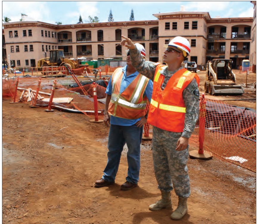
Cadet Calvin Kiesewetter (right) asks Construction Control Representative Joe Tribbey about a window frame at the Corps' Quad B renovation project site. Photo by Dino W. Buchanan
