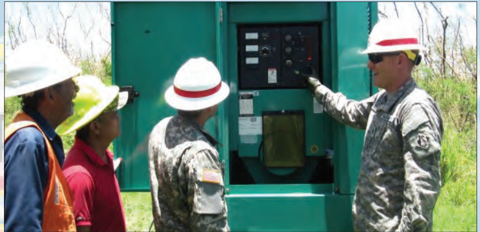
In support of the governor, local responders, the Federal Emergency Management Agency (FEMA), and a USACE Power Planning and Response Team (Power PRT) from the Honolulu District made a huge difference. This specialized team worked with the U.S. Army's 249th Engineer Battalion, contractors, and commonwealth and local entities to assess, install and maintain emergency generators at critical facilities, especially at wells to ensure that residents of Saipan get a much-needed supply of drinking water. Courtesy photos
