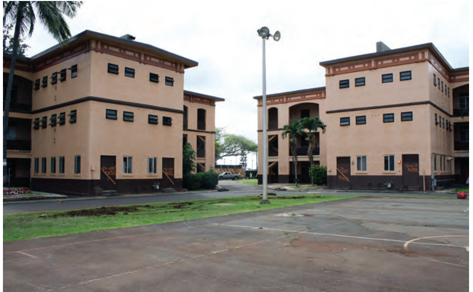
Buildings 158 (left) and 157 in Quad B at Schofield Barracks are two of the facilities being renovated. Building 158 was built in 1914. Photo by Dino W. Buchanan
