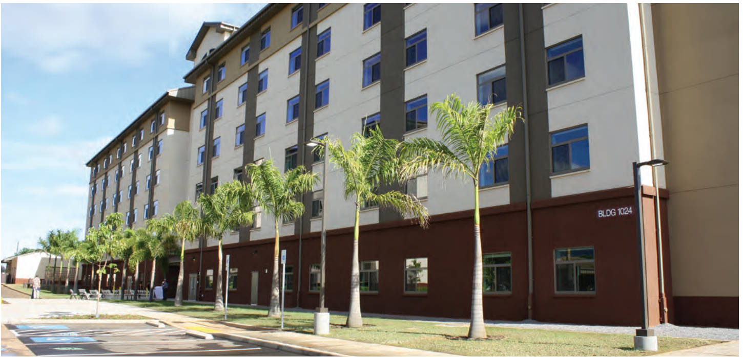
The U.S. Army Corps of Engineers, U.S. Army Garrison-Hawaii and contractor Absher Construction officials opened the new $35.3 million barracks during a ribbon-cutting ceremony Oct. 30. The six-story Unaccompanied Enlisted Personnel Housing on Montague Street houses Soldiers of Headquarters and Headquarters Battalion, 25th Infantry Division and the 2nd Brigade. Photo by Dino W. Buchanan
