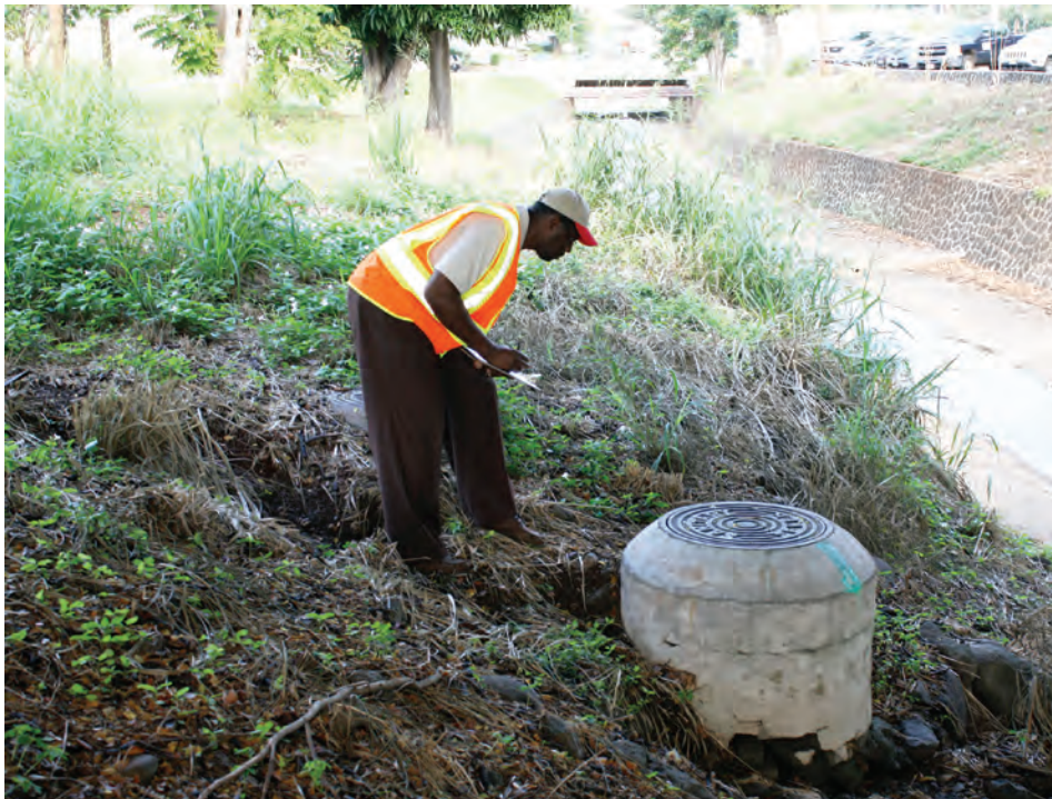
Keith McDonald analyzes a manhole cover and cement casing for deterioration and cracks during a facilities data collection inspection on Fort Shafter. Photo by Dino W. Buchanan
