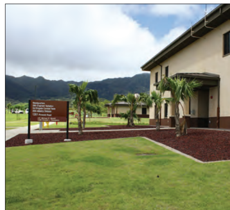
The 29th Engineer Battalion Headquarters was one of the new facilities built by the Corps of Engineers on the South Range Road Project cantonment. Photo by Dino W. Buchanan
