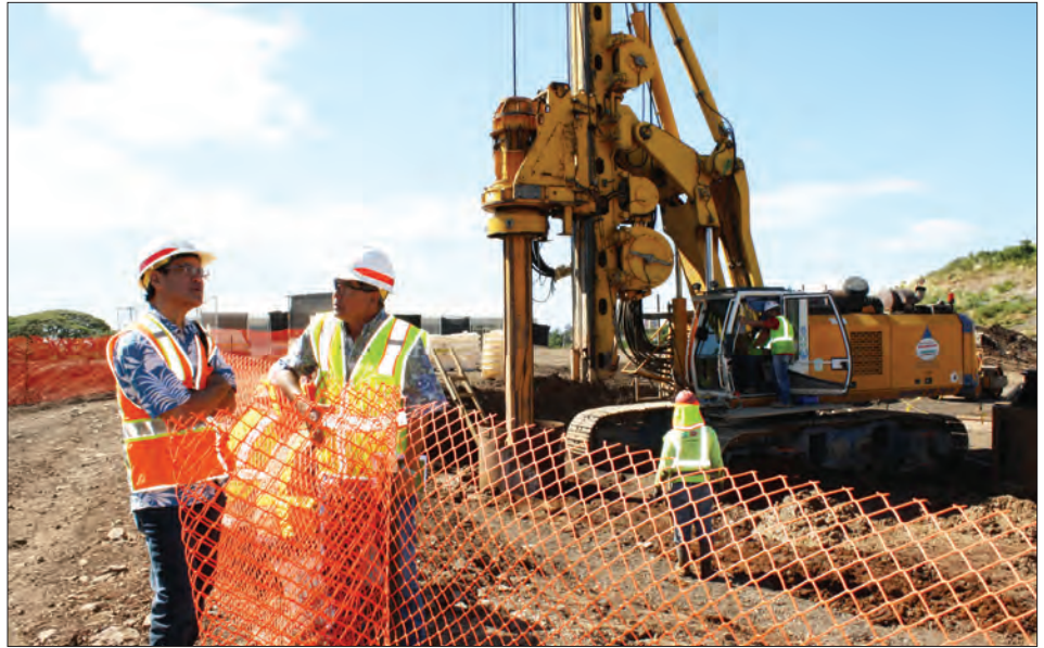
Project Engineer Gerald Young and Construction Control Representative Scott Mochizuki discuss a caisson drilling process on the MCF Contract 2 site in January. Photo by Dino W. Buchanan
