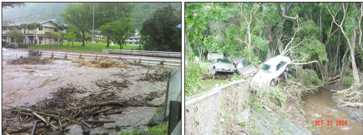
Figure 2. October 2004 Flood, Debris Blockage and Car Damage at Woodlawn Bridge, Mānoa Stream
