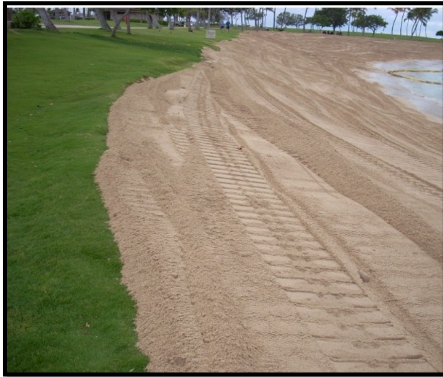
Figure 2-21 Beach face after grading
