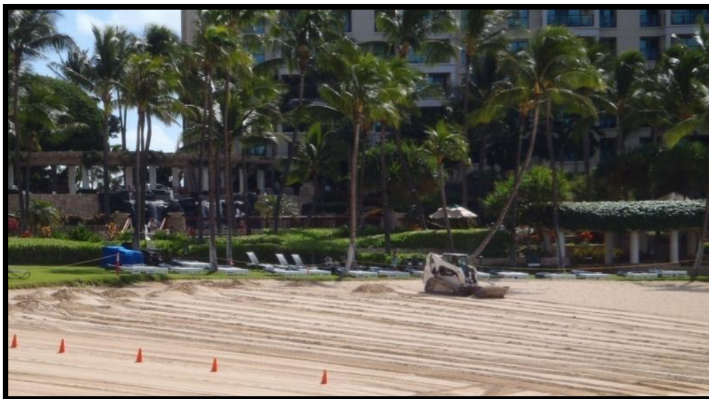
Figure 2-23 Bobcat pulling sand upslope on the beach profile
