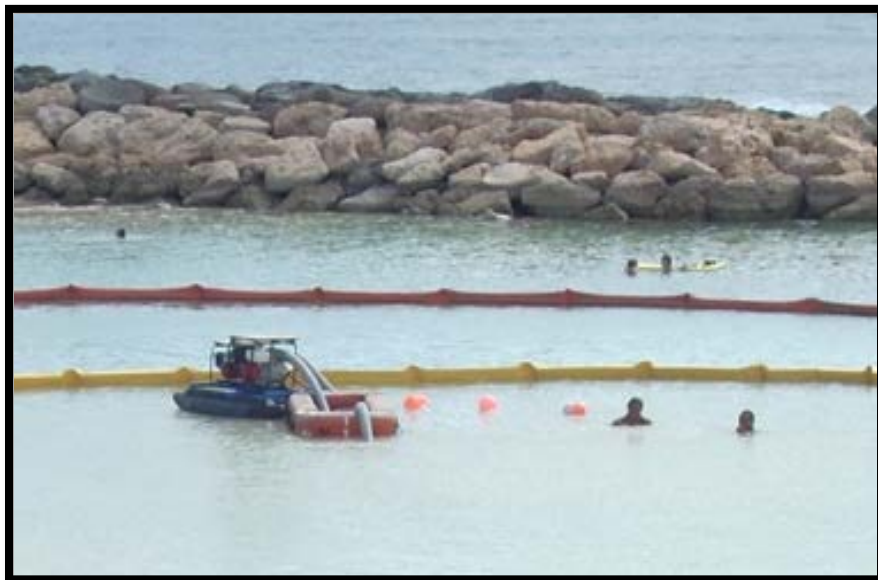
Figure 2-5 Piranha PS165-E dredge system deployed at Ko Olina
