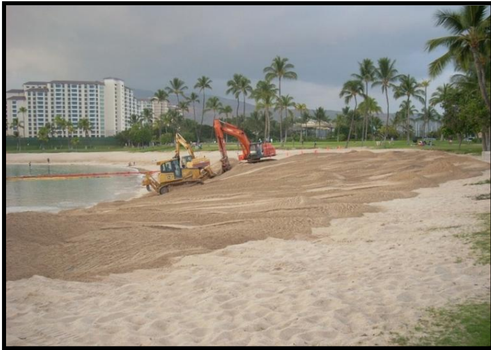
Figure 2-11 Heavy machinery working on the beach, double sit curtains deployed
