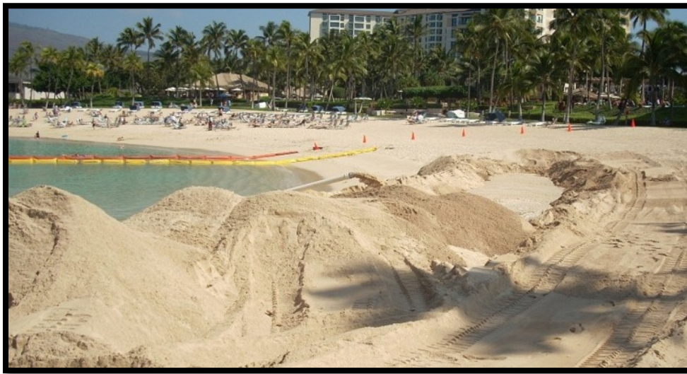
Figure 2-19 Typical discharge pipe and dewatering basin setup
