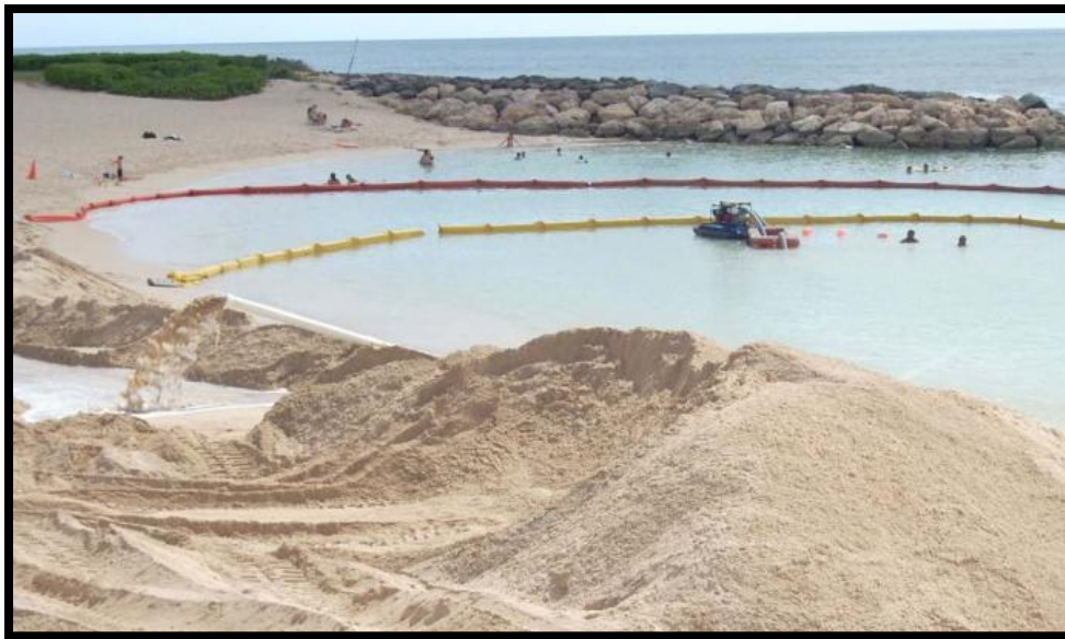
Figure 2-17 Suction dredge and dewatering operations using the Piranha 165E, double sit curtains deployed
