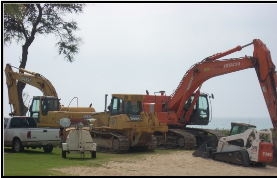
Figure 2-8 Typical staging area for heavy equipment
