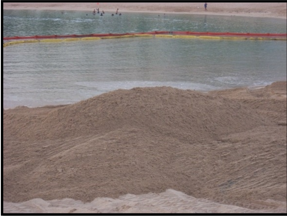
Figure 2-20 Beach face after sand moving, prior to grading
