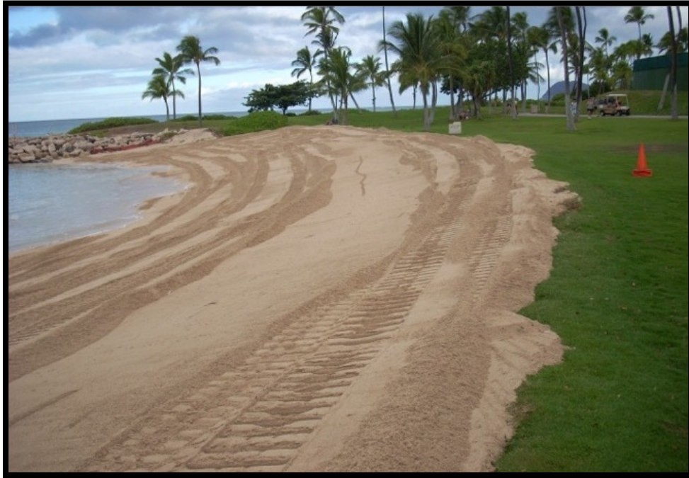
Figure 2-13 Beach face after grading
