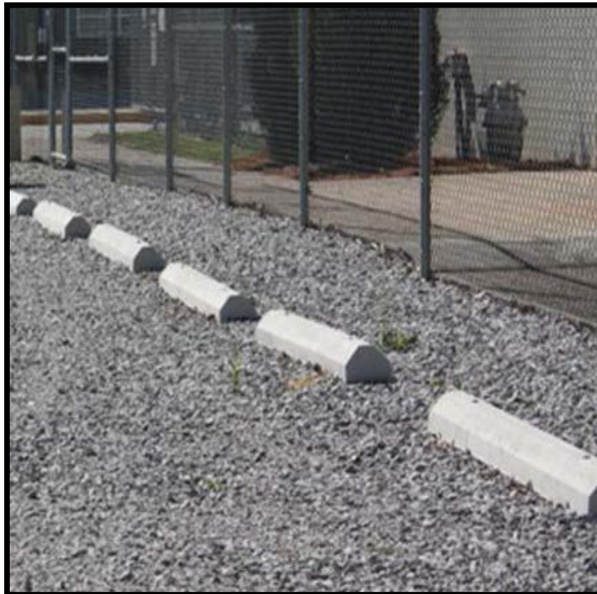
Figure 1-6 Typical parking lot wheel stops
