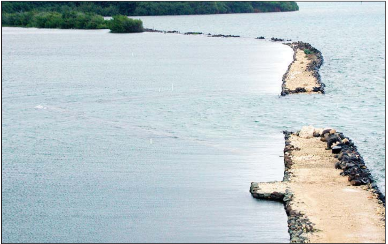
Figure 8. Submerged Temporary Wall and makai fishpond wall with break looking north at high high tide, 2.8 ft. (6/17/2011).
