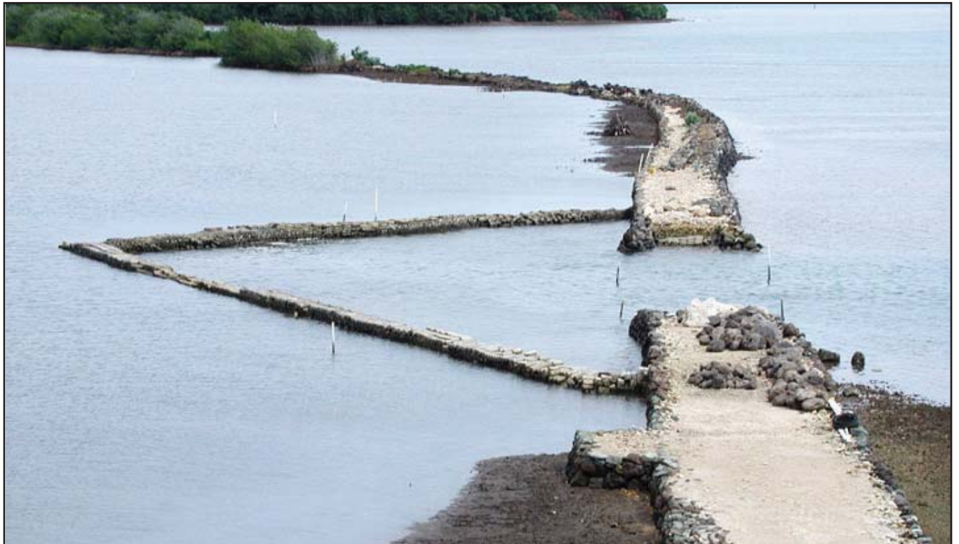
Figure 9 Same view at low low tide, -0.10 ft. (4/8/2011). The Temporary Wall is 3 ft. high and 3 ft. wide; The north wall segment is 95 ft. long, and south wall segment is 158 ft. long.
