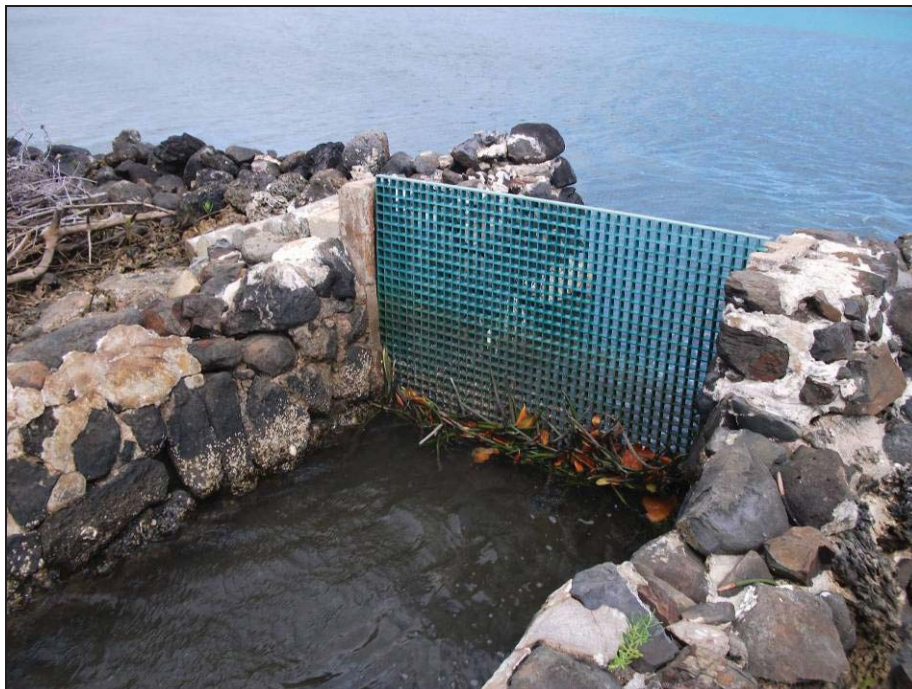
Figure 27. Mākāhā north of Makai Break; note use of concrete to maintain kuapā , view to northeast
