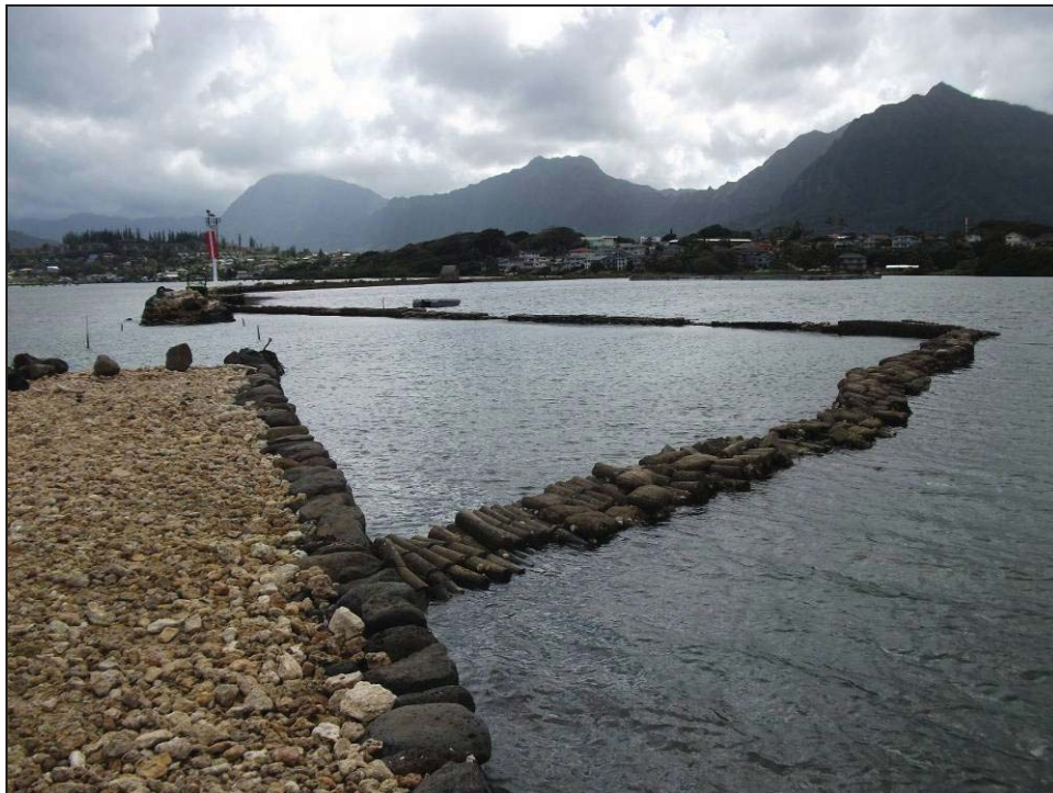
Figure 23. Detail of cement-cylinder wall mauka of break, view to southwest
