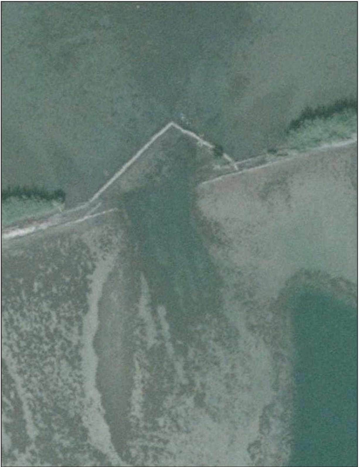
Figure 7. Aerial Photograph - Project Site - Makai Wall Break He'eia Fishpond, Kāne'ōhe Bay, He'eia, Ko'olauloko, O'ahu (Photo: Google Earth cir. 2007).
