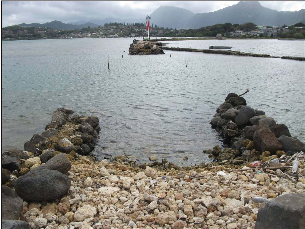
Figure 20. Looking across the Makai Break; a portion of temporary wall is visible to the right, view to south
