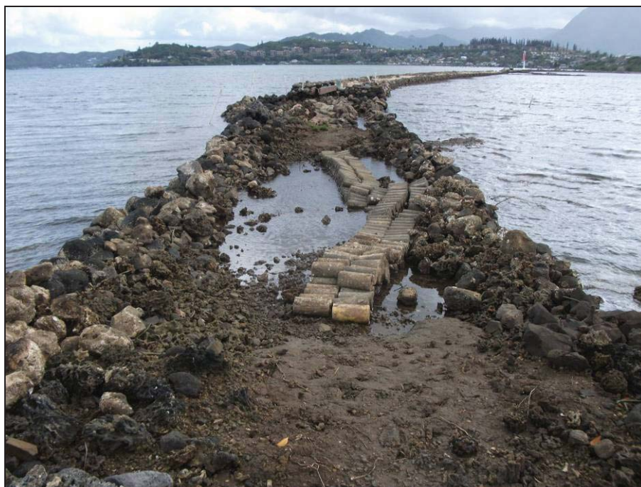
Figure 29. Photograph showing makai portion of kuapā where mangrove has been removed. Note the extent of damage to the kuapā from the mangrove and the use of cement cylinders as fill, view to south; the Makai Break is to the southwest
