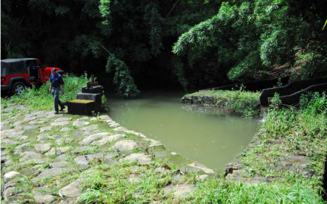
Figure A8: Stream diversion into the Center Ditch downstream from reservoir, March 2010
