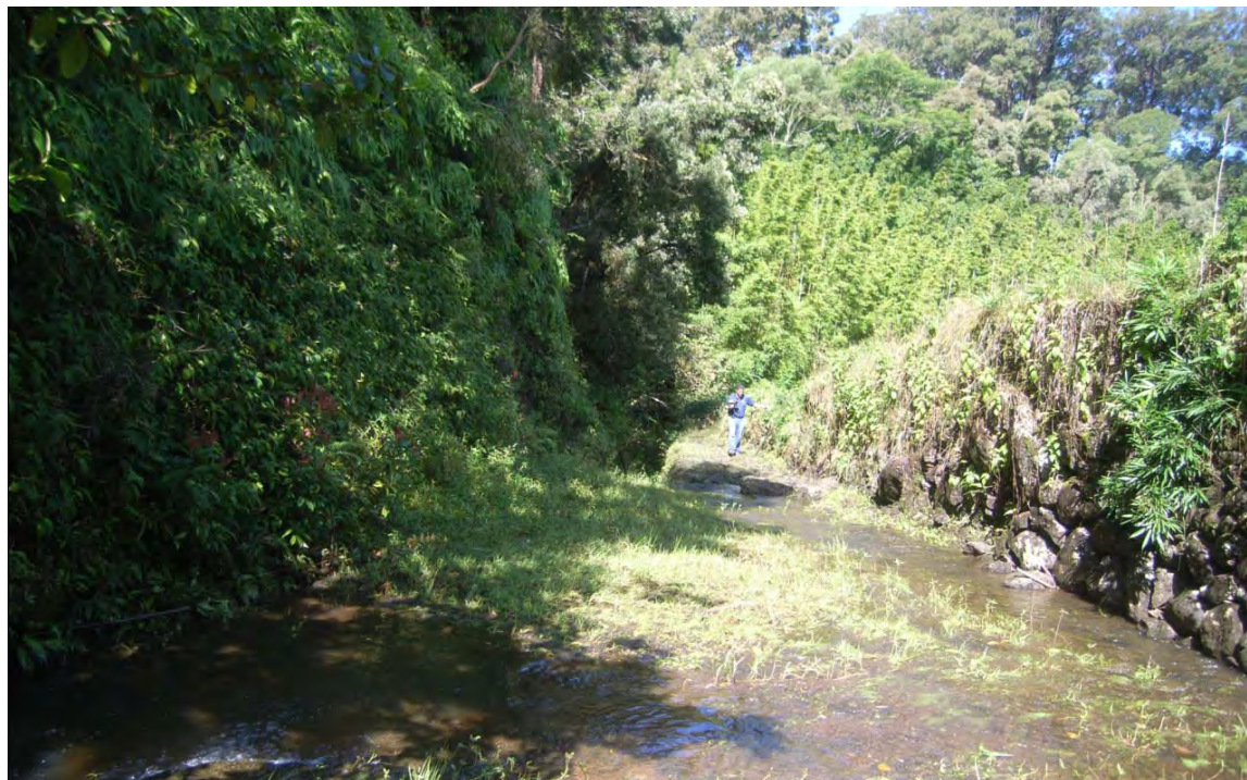
Figure A7: Kolea Reservoir spillway looking downstream, March 2010
