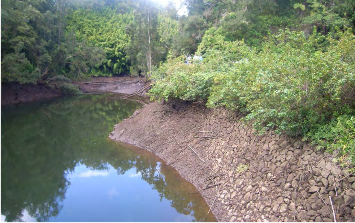
Figure A2: Kolea Dam upstream face riprap looking upstream, September 2009
