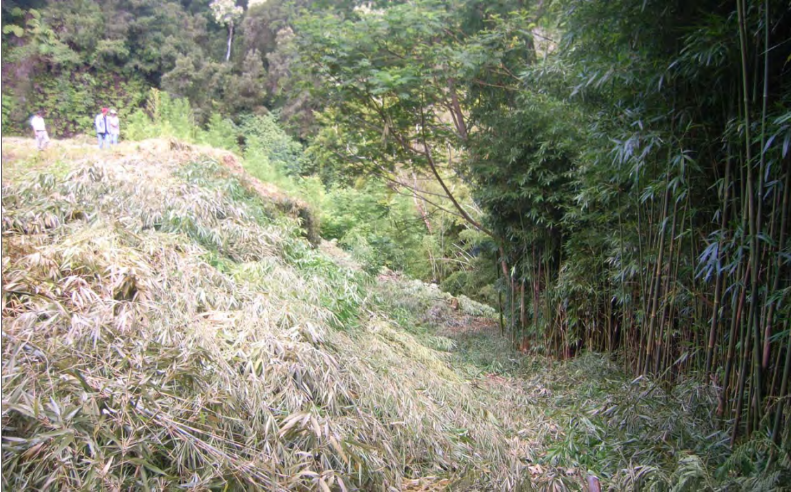
Figure A4: Kolea Dam downstream face looking upstream, September 2009
