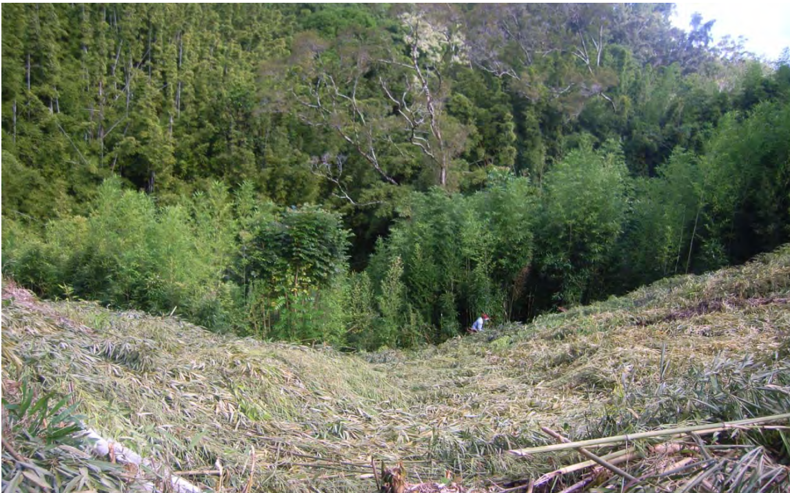
Figure A5: Kolea Dam downstream face looking downstream, September 2009
