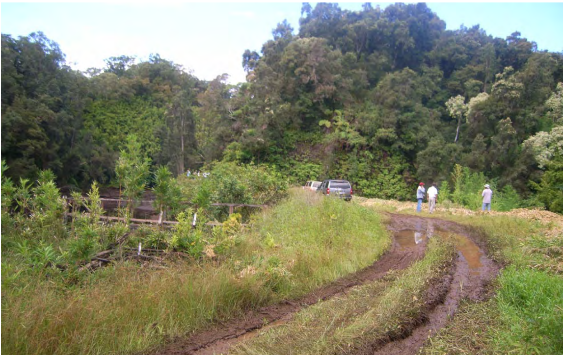
Figure A3: Kolea Dam crest and access road looking upstream, September 2009
