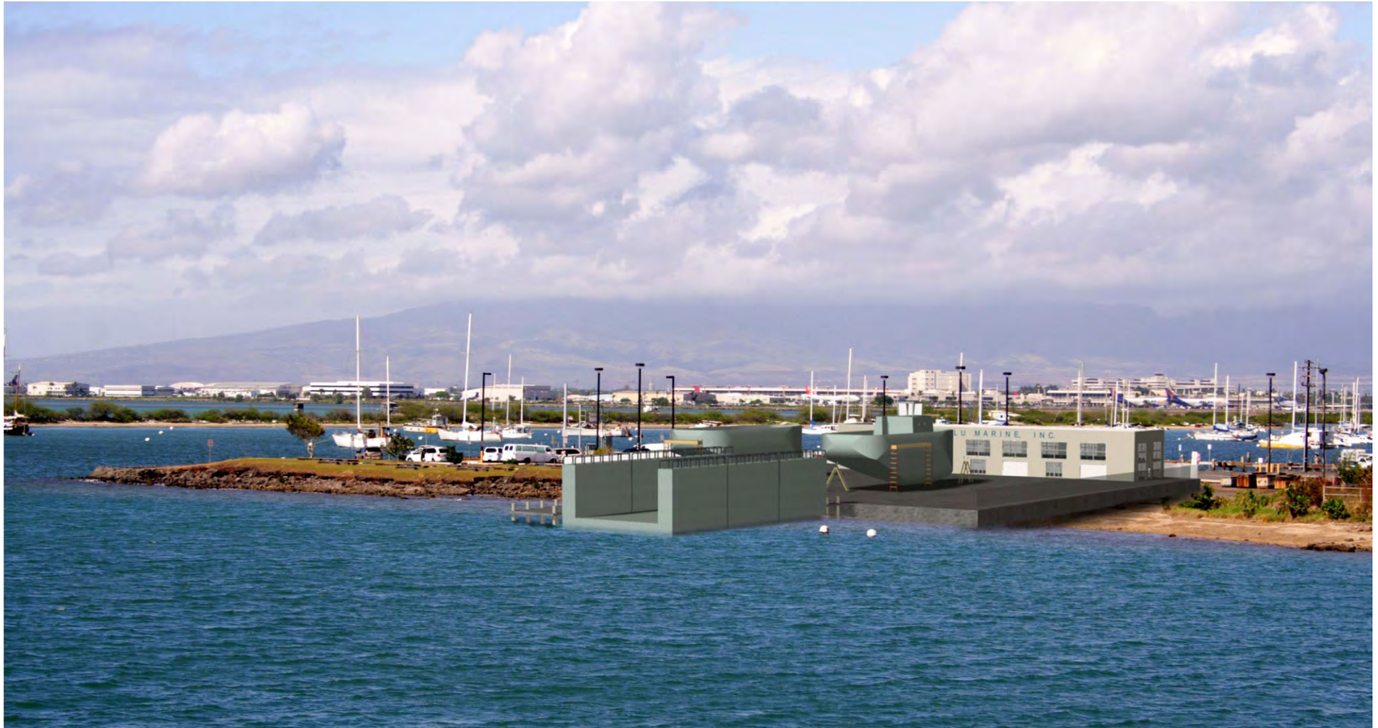
View from Bridge Facing West
