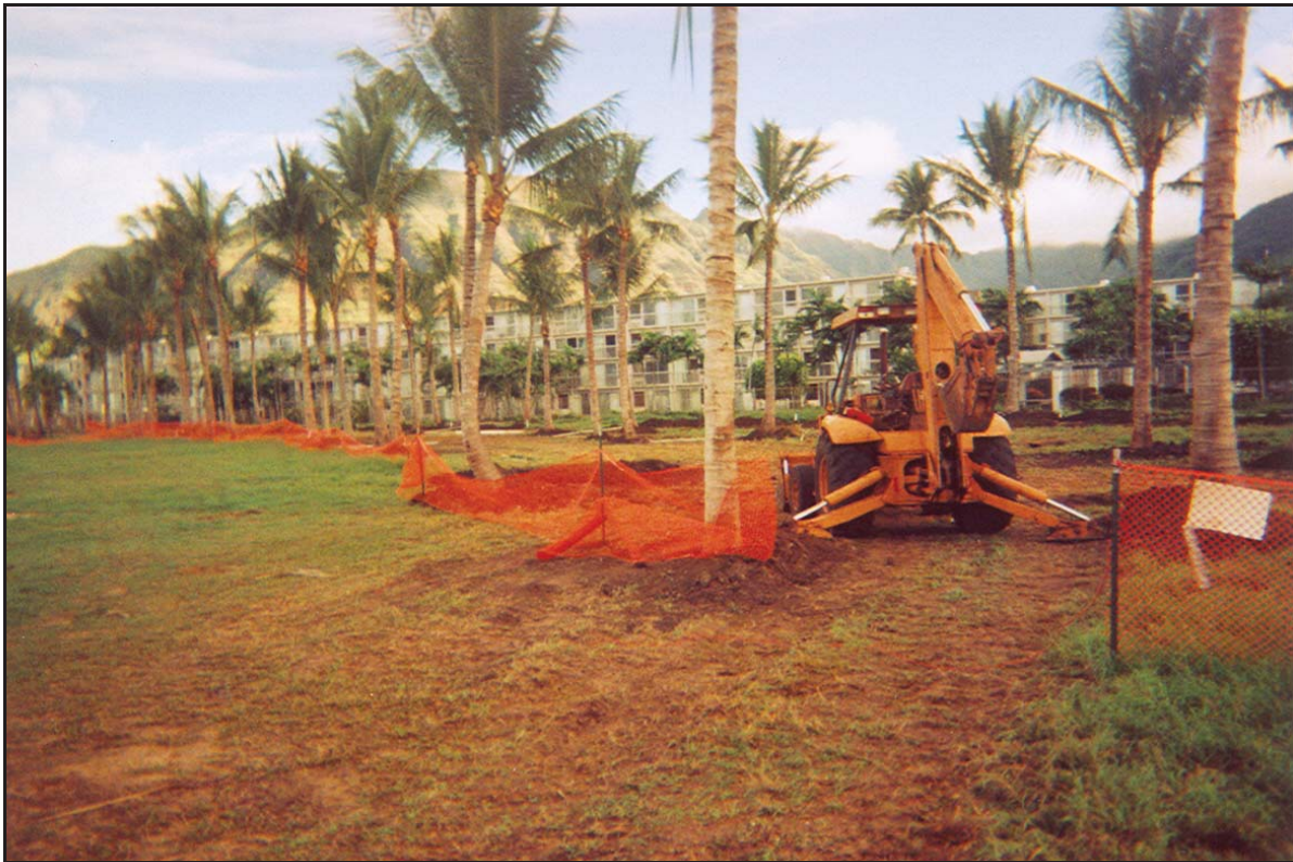
Figure 3. Photograph of preventive construction fencing, view to northwest
