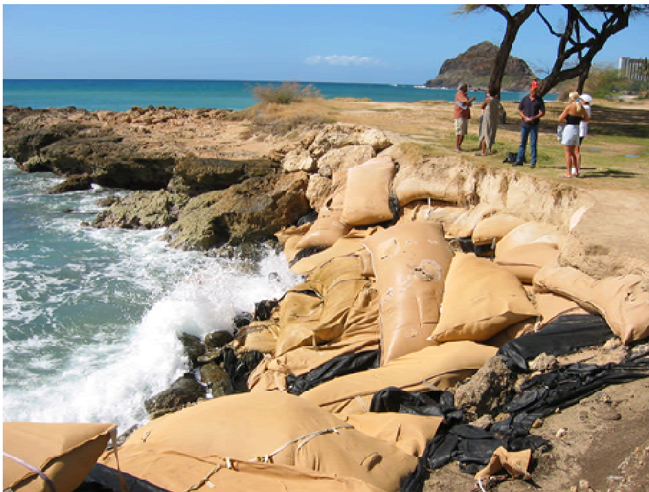
Damage to Sandbag Protection from Waves Entering Breakwater Gap (Jan 19, 2006)
