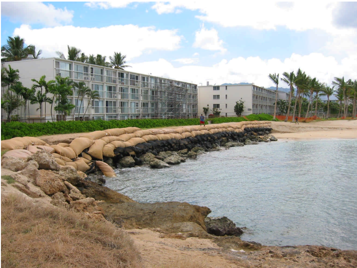
Figure 1. Existing Sandbag Revetment
