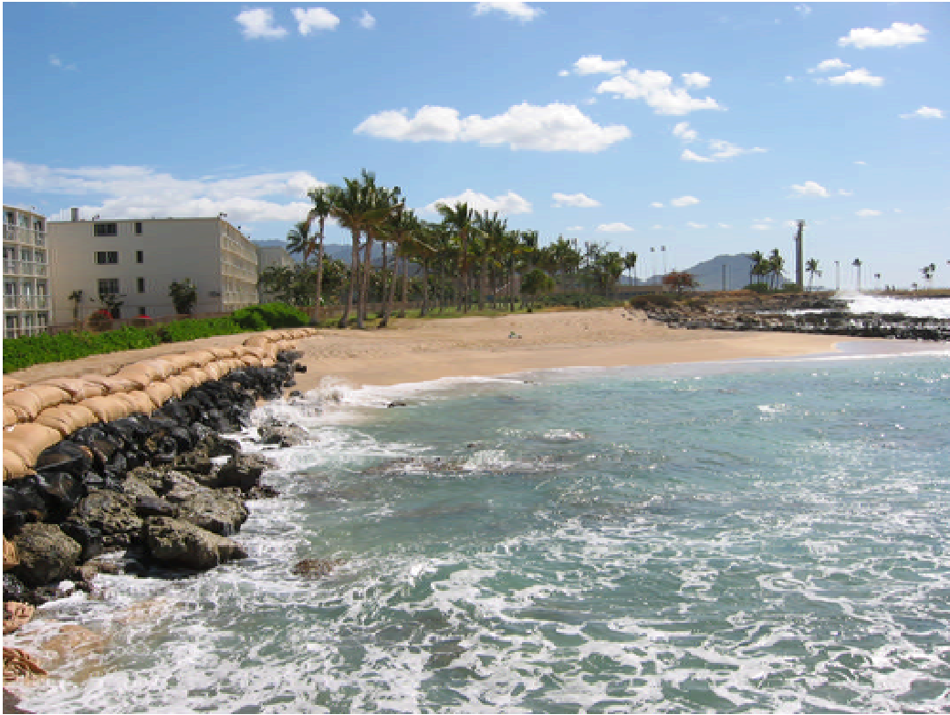
Sandbag Revetment and Beach at South End of Cove
