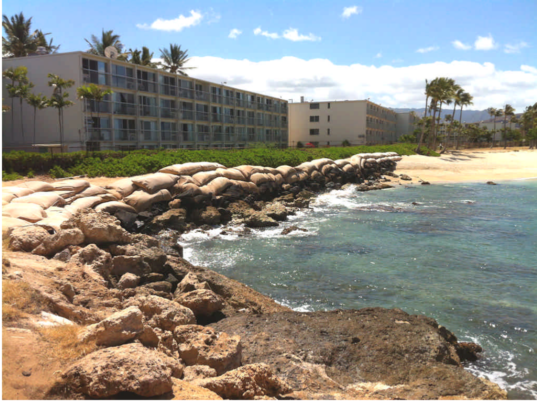
Figure 3. Existing Sandbag Revetment Fronting Makaha Surfside
