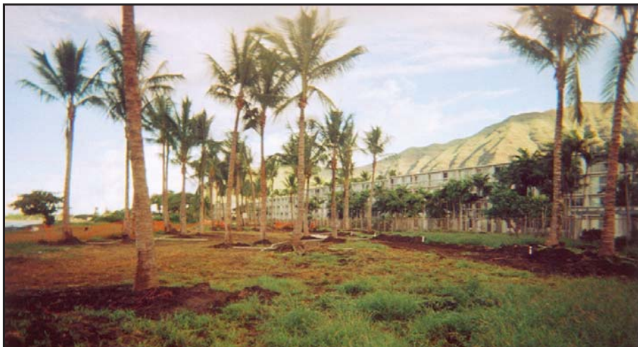
Figure 7. Photograph of the construction fence boundary (the orange fence is visible at the left side of the image) showing the excavations contained within the mauka half of the project area, view to northwest.
