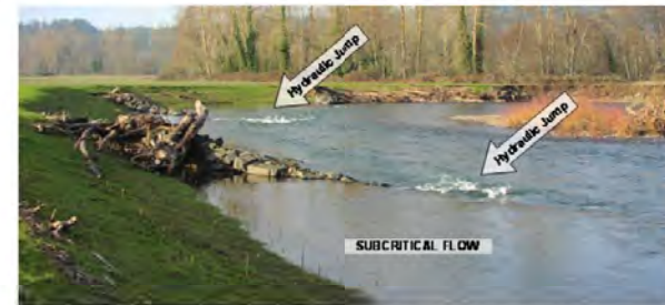
Figure 7. Hydraulic effects across and upstream of stream barbs at intermediate discharge.
