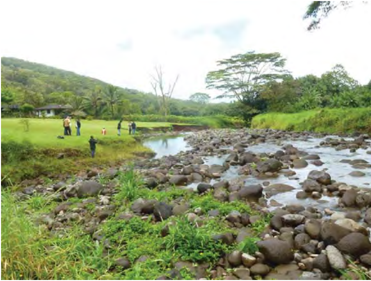
Photo 5. The run-off flow through the breach already eroding the streambank while moving laterally towards adjacent residents.
