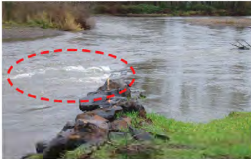
Figure 5. Turbulent zone at intersection of cross-structure flow and contraction accelerated flow at 75% bankfull discharge.
