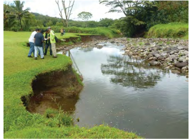
Photo 6. Closer view of the area shown in Photo 5. Run-off flow through the breach eroding the streambank while moving laterally towards adjacent residents.
