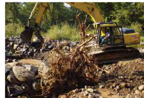
Figure 9. Large wood placement within barb section.
