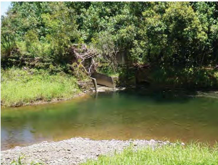
Photo 7. Intake pipe located upstream of the point of re-entry of the breach water to the stream that feeds the water for Hanalei taro farms and the USFWS refuge grounds.
