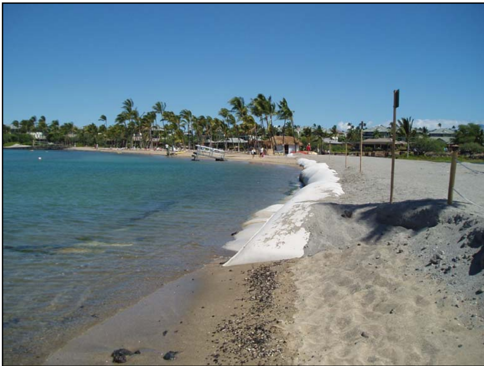
Figure 1-7 Temporary Repairs in the Tsunami Breach at Waikoloa Beach, as Photographed 20 September, 2011
