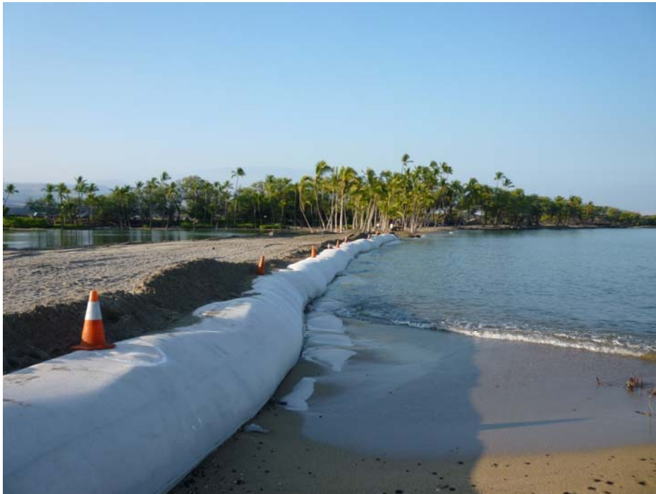
Figure 2-3 Post Emergency Repair, August 4, 2011
