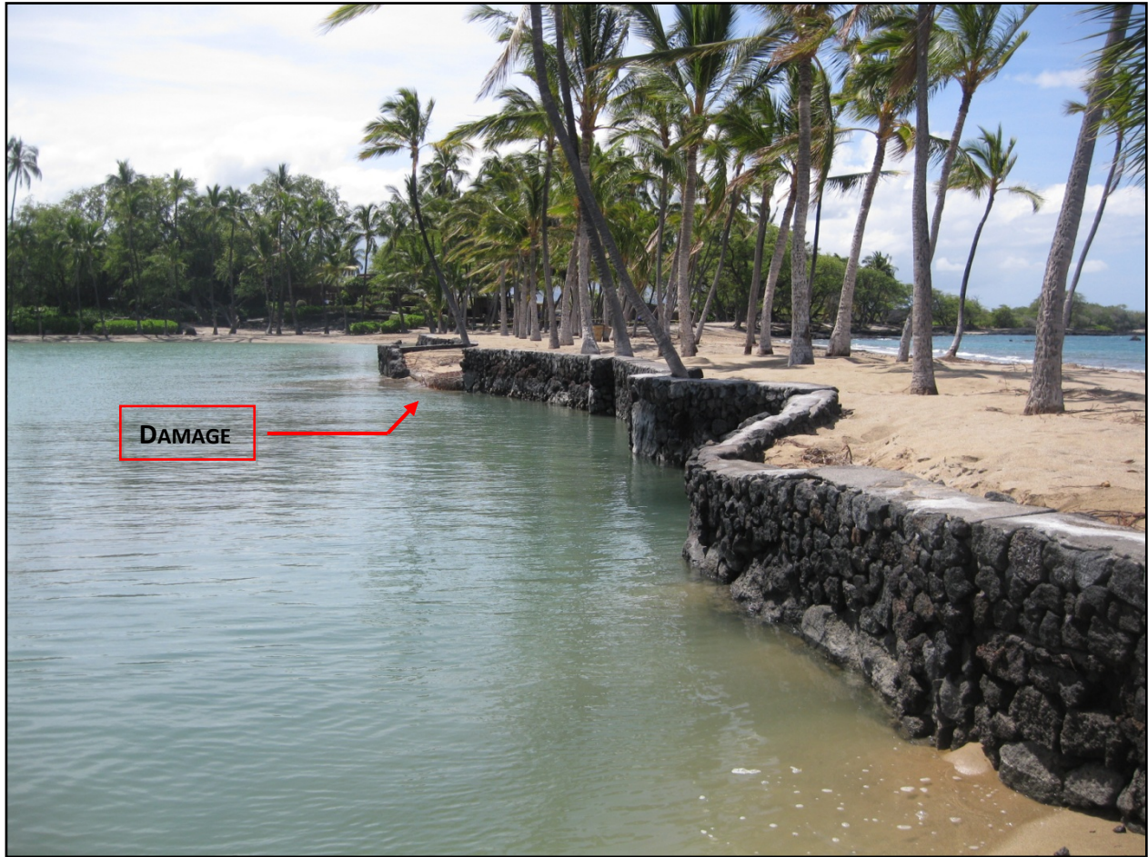
Figure 3-1 Existing Pond Wall
