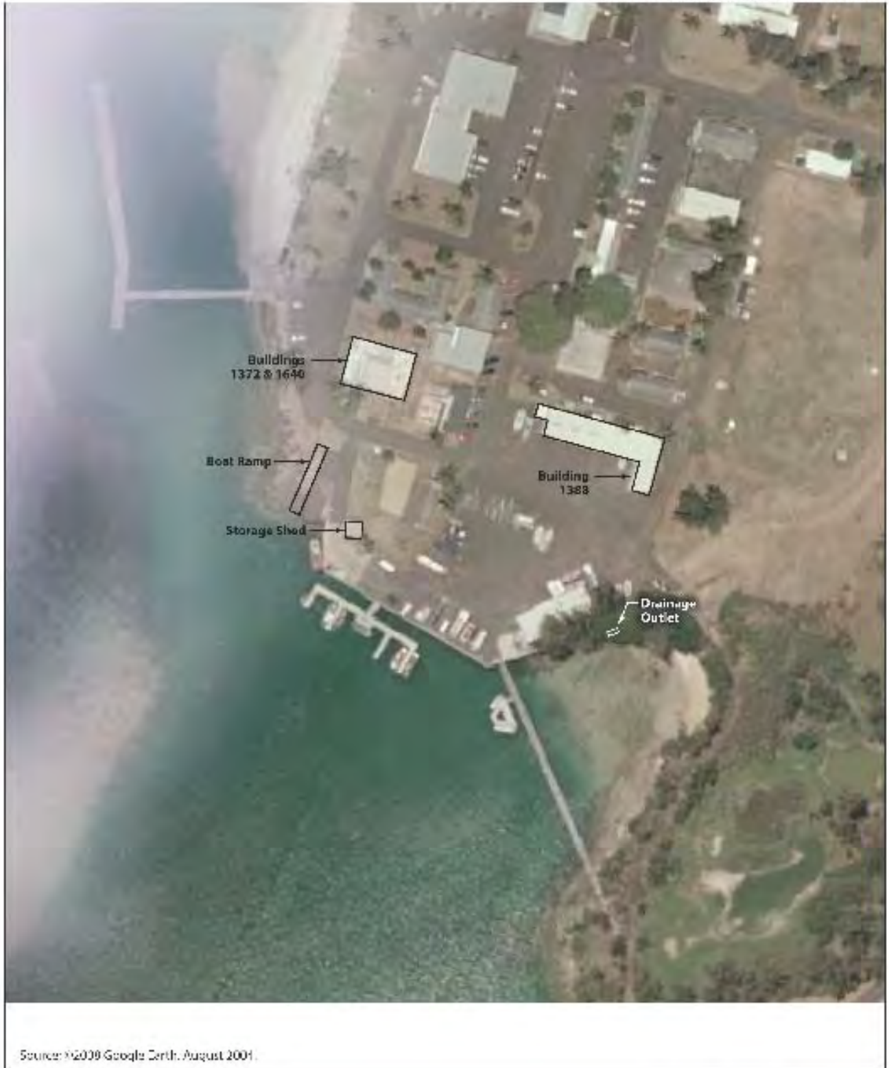
Figure 2 AERIAL VIEW OF WFO SITE SHOWING AFFECTED STRUCTURES
