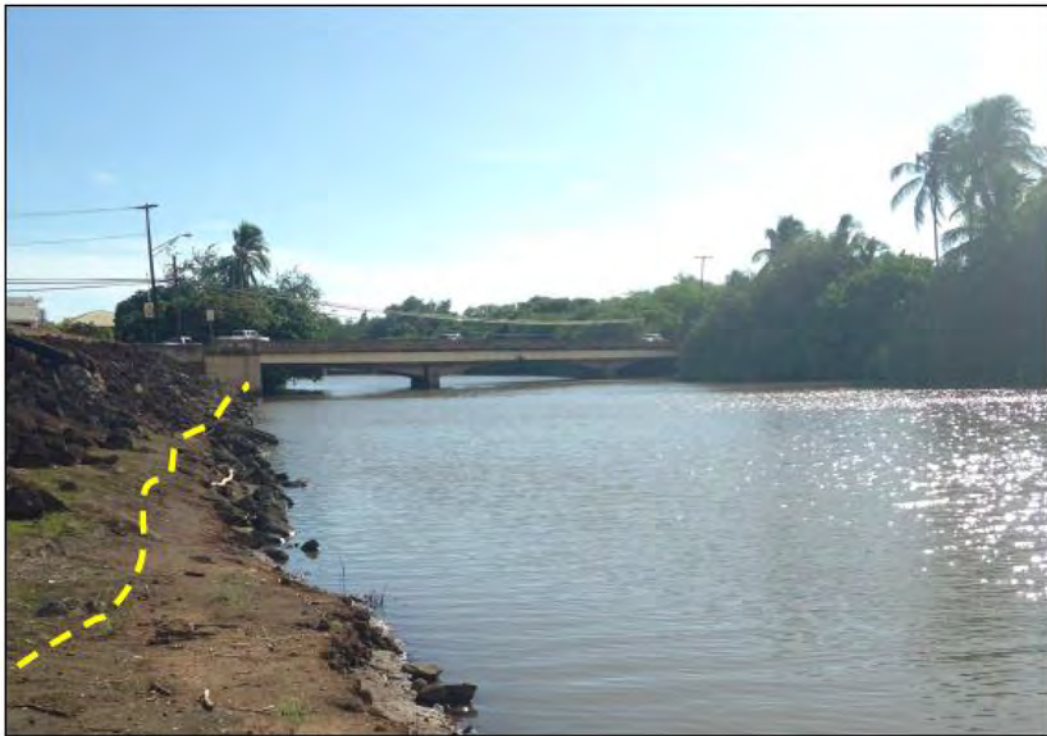
HANAPEPE RIVER BRIDGE, SHOWING MODIFICATIONS ON THE RIGHT BANK.
