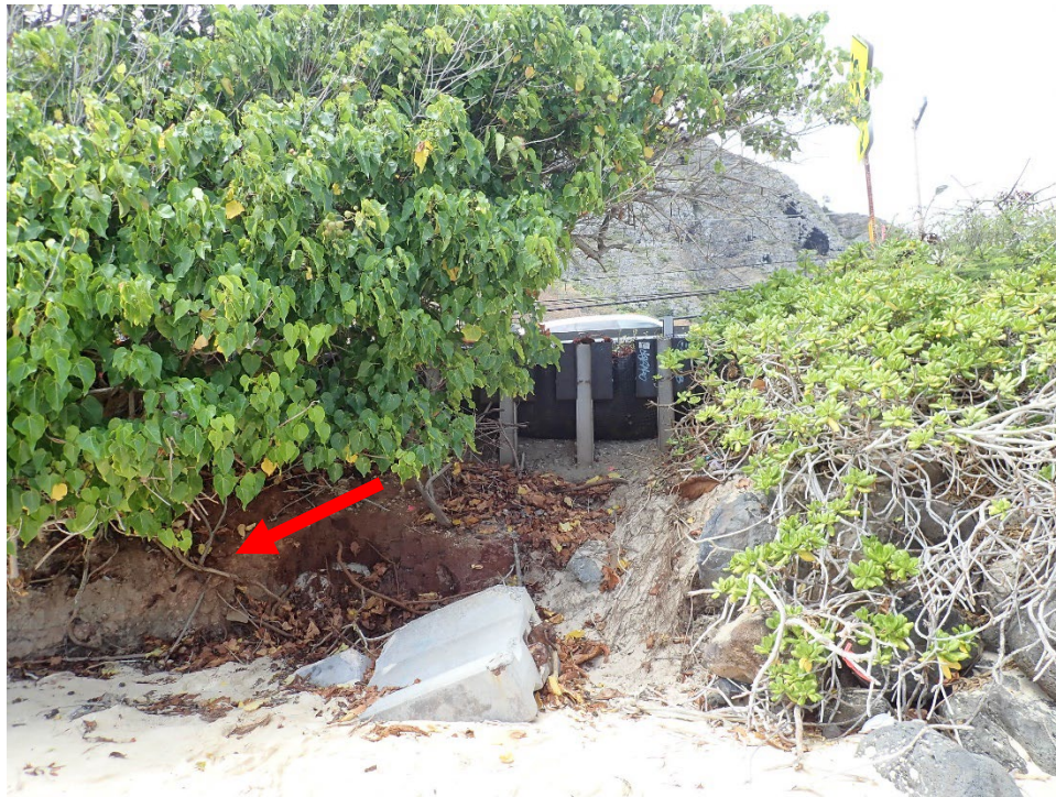
Photo 6-3: Culvert Outlet Buried and Broken
