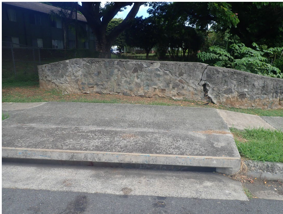
Above: Looking downstream from Kakaina St (headwall does not tie into high ground)
