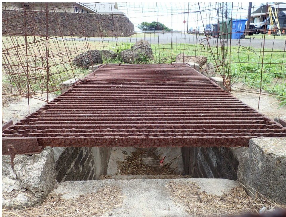
Photo 2-15: Intake / Culvert Inlet along Bell Street
