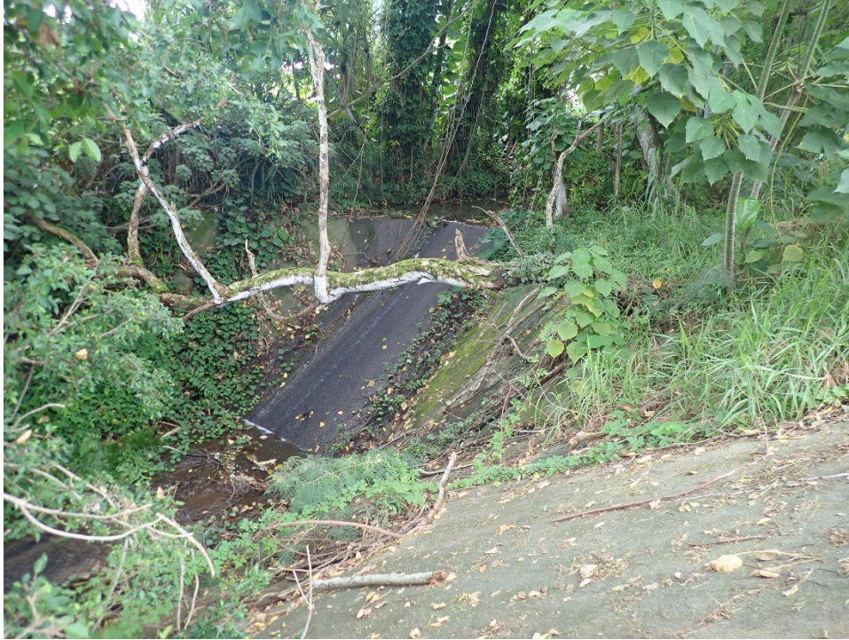
Above: Weir and drop structure located upstream of Waikupanha Culvert 1
