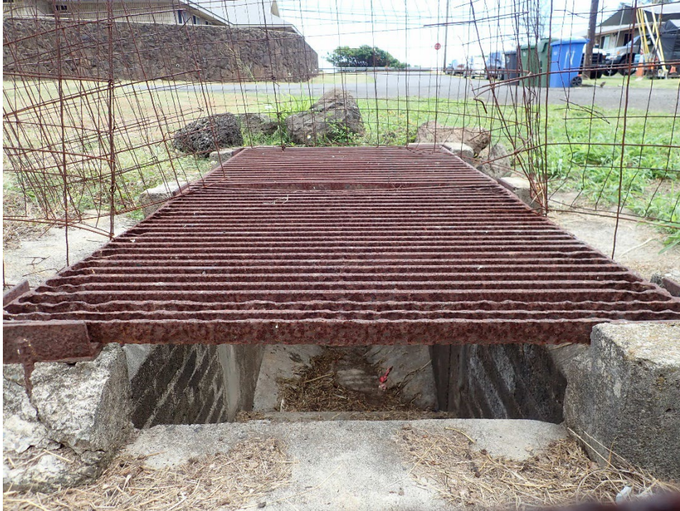
Photo 6-2: Intake / Culvert Inlet along Bell Street
