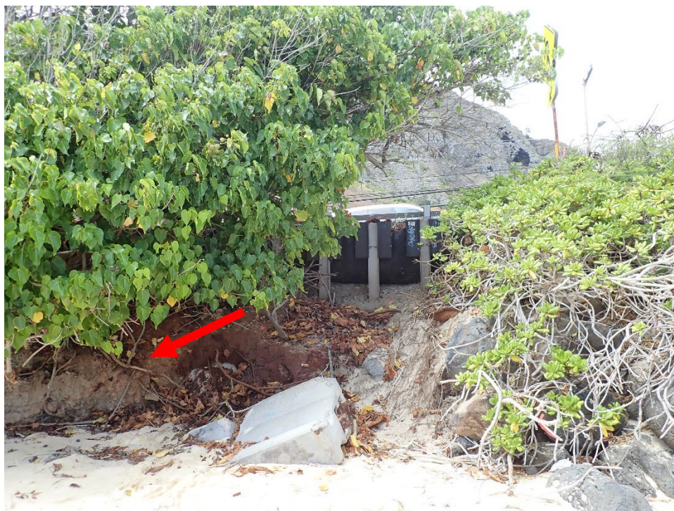
Photo 2-16: Culvert Outlet Buried and Broken
