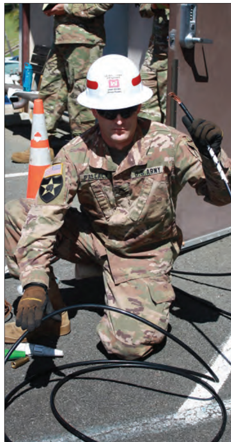
During the training Staff Sgt. Jason Pallack conducts an inspection of the cable terminations prior to connecting a generator to the affected facility during the 249th Engineer Battalion training exercise at Honolulu District. Photo courtesy of Pacific Ocean Division
