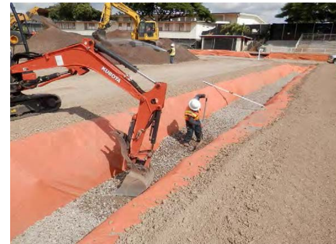
Photo 3: Select borrow (clean fill) placed on top of geofabric liner
