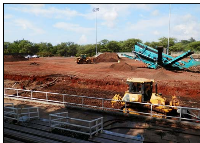
Photo 1: Excavation and mechanical screening at RHS track
