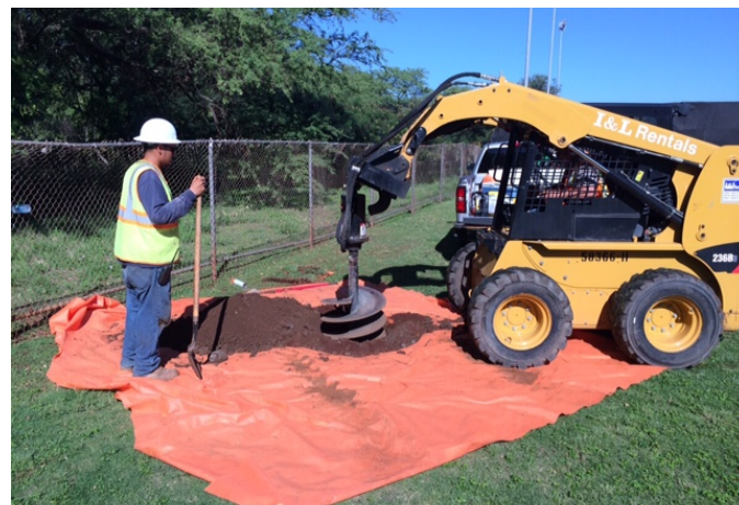
Photo 5: Drilling test pit borings at RHS baseball field
