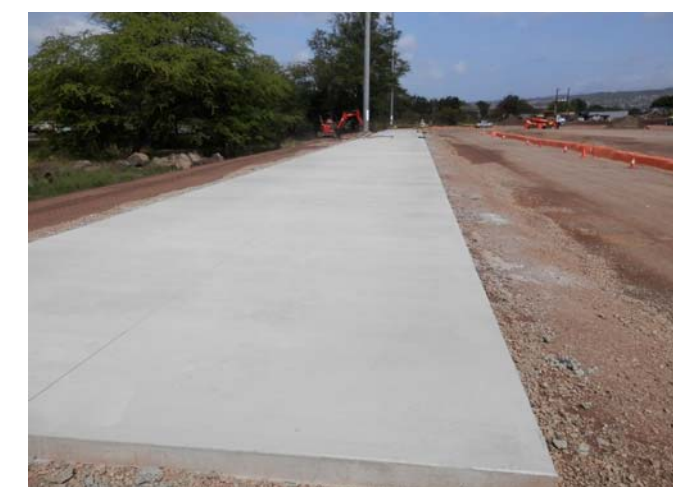
Photo 4: Slope stabilization and concrete cap
