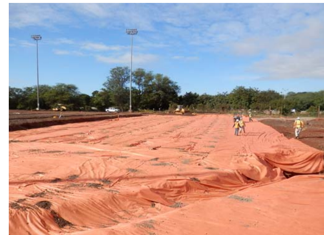
Photo 2: Geofabric liner installed prior to placing clean fill
