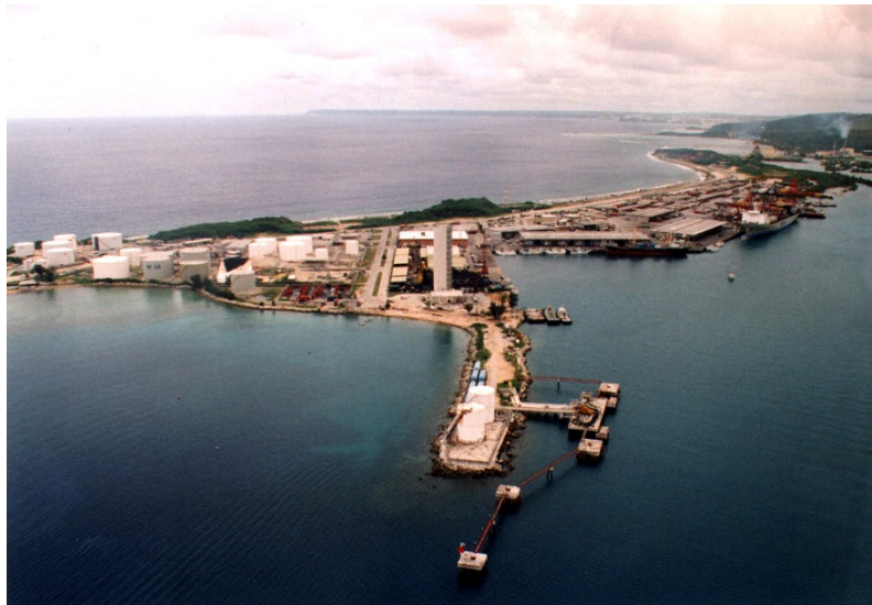
F-1 Fuel Pier at Guam
