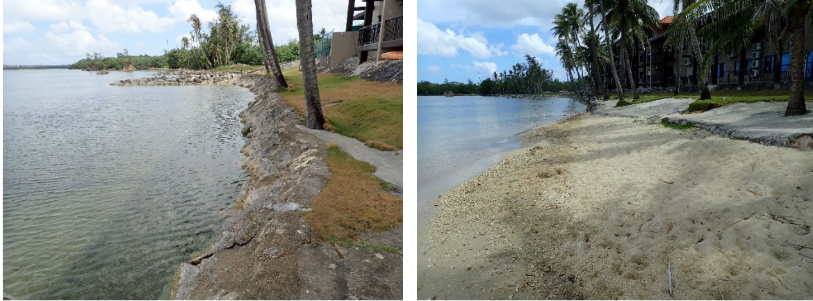
Figure 71. Inn on the Bay property, looking north. Typical of northern section on the left, with no beach fronting the wall. Typical southern section on the right, where a sandy beach starts to form.
