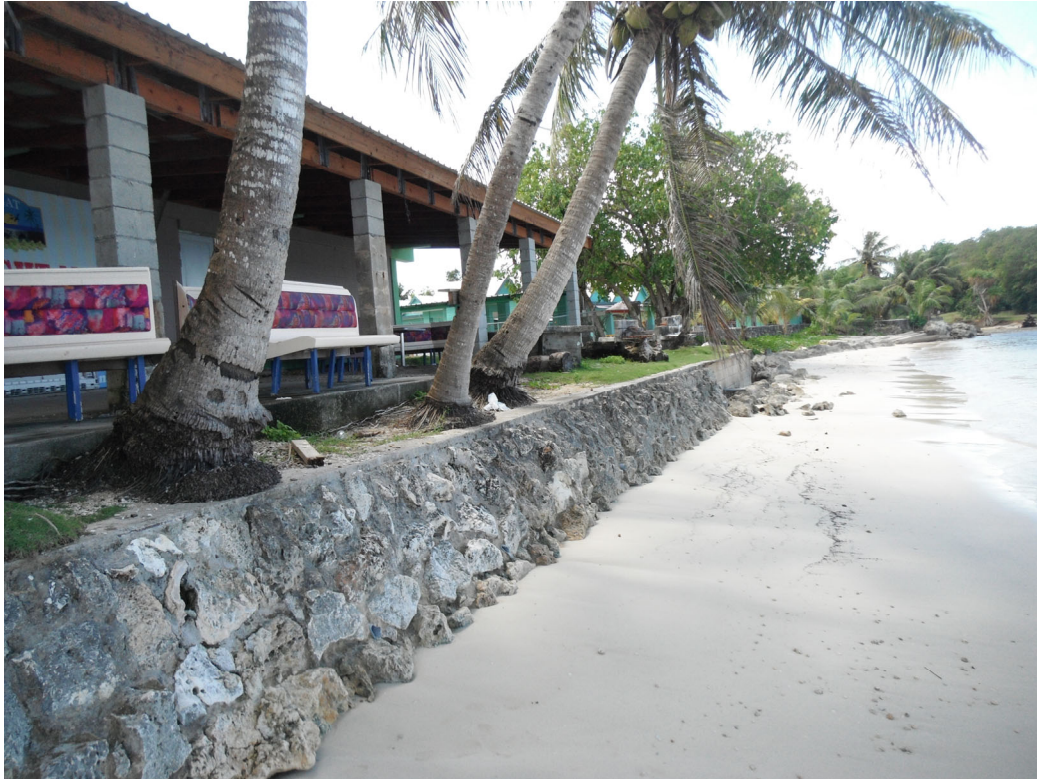
Figure 77. Grouted CRM wall protecting Agat Mayor's Office in the foreground. Teal pavilions in the background are part of Agat Sagan Bisita.
