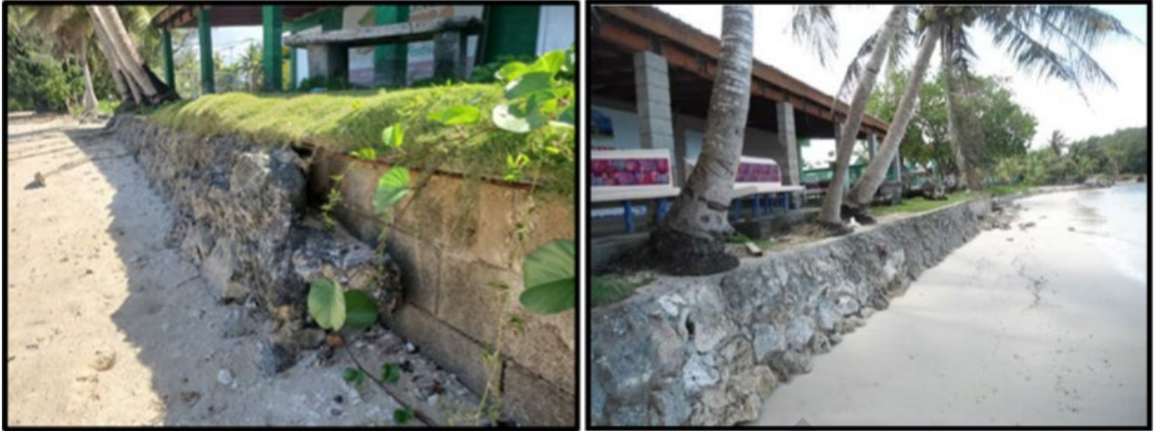
Figure 3: Undermining of the existing seawall fronting the Community Center.
