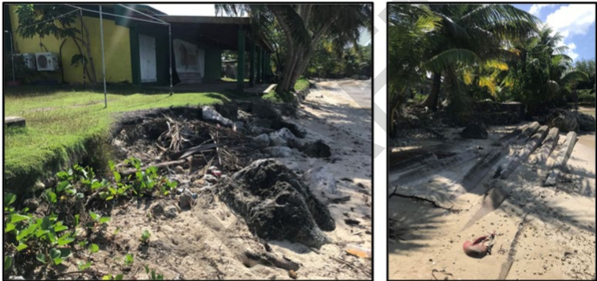
Figure 4: Large rocks and utility poles for temporary protection to the Community Center and Sagan Bisita.
