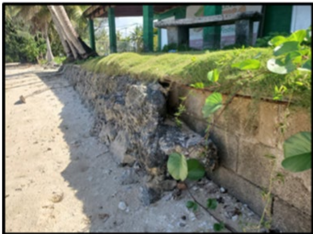
Figure 10: Undermining of the existing seawall fronting the Community Center. Image source: USACE, January 2022
