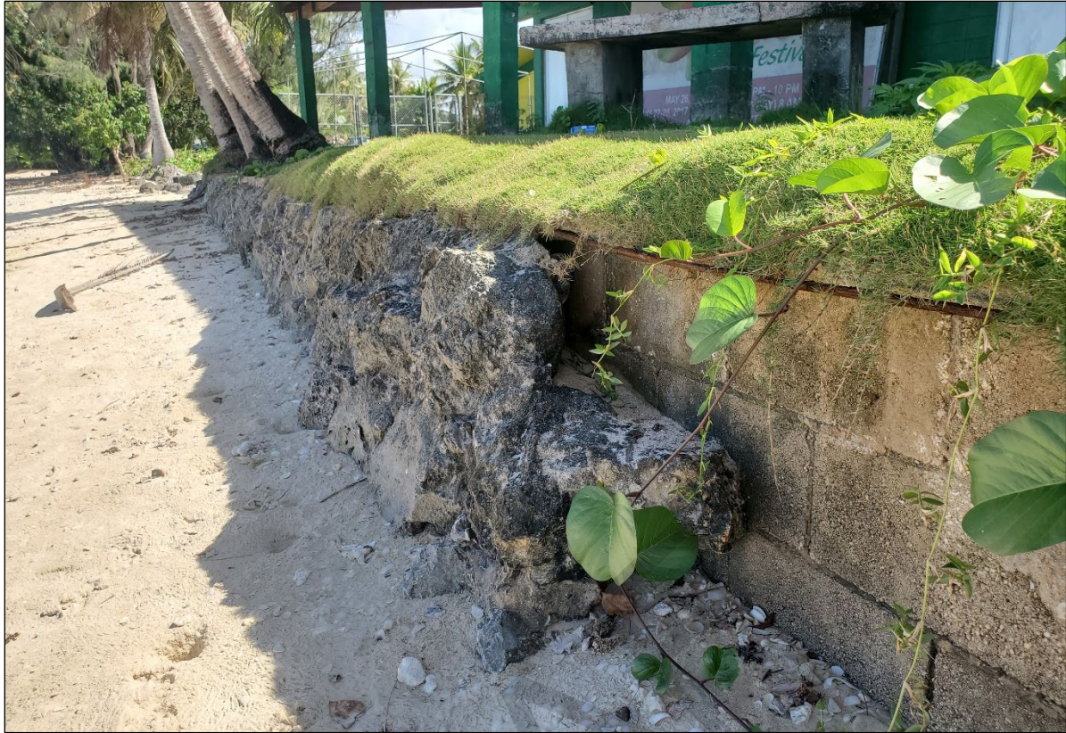
Figure 2. Existing seawall along the Agat shoreline; damaged rock and brickwork visible.
