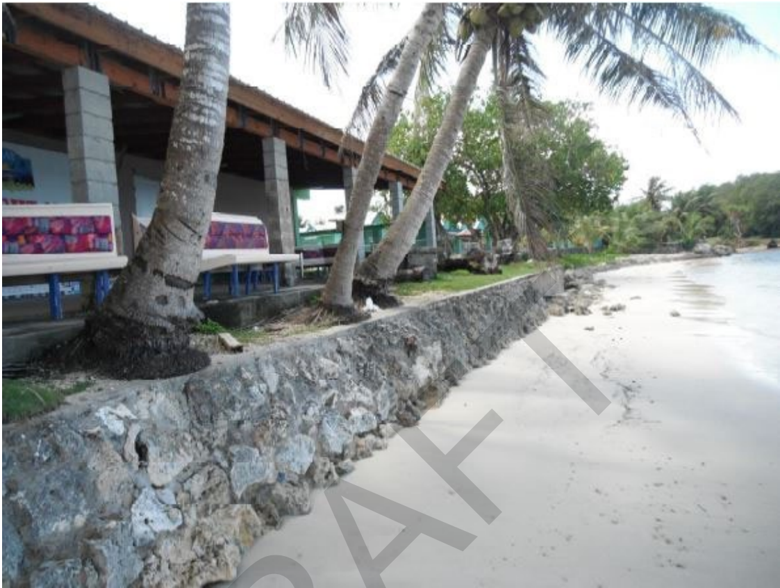
Figure 4. Rock masonry wall, infrastructure, and shoreline threatened by erosion (Image provided by USACE).
