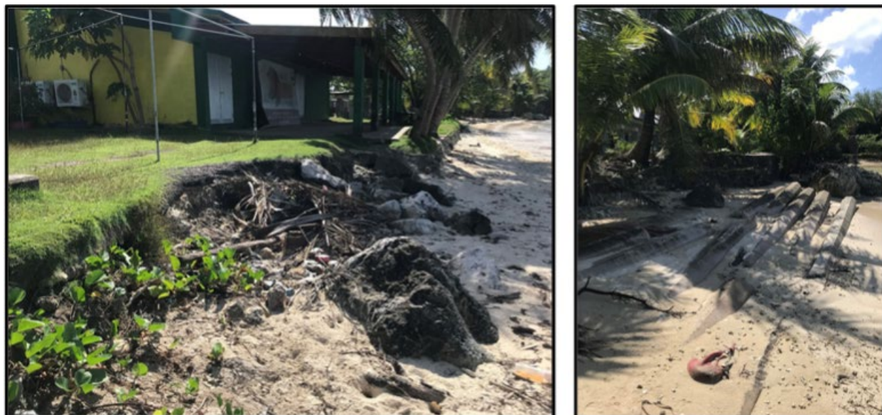
Figure 11: Large rocks and utility poles for temporary protection to the community center and Sagan Bisita. Image source: USACE, January 2022
