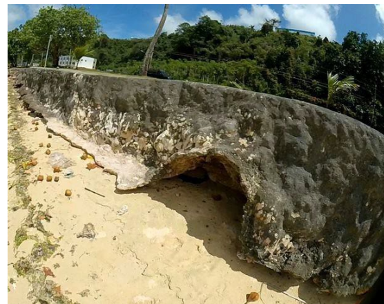
Figure 5. Voids where wall was constructed around trees that have since been removed or fallen
