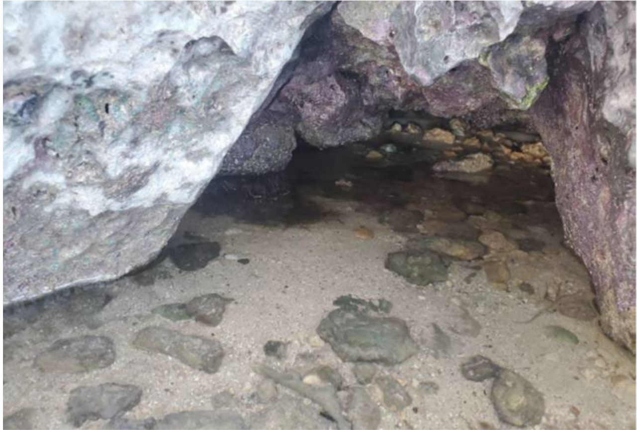
Figure 2. Undercutting of Existing Wall
