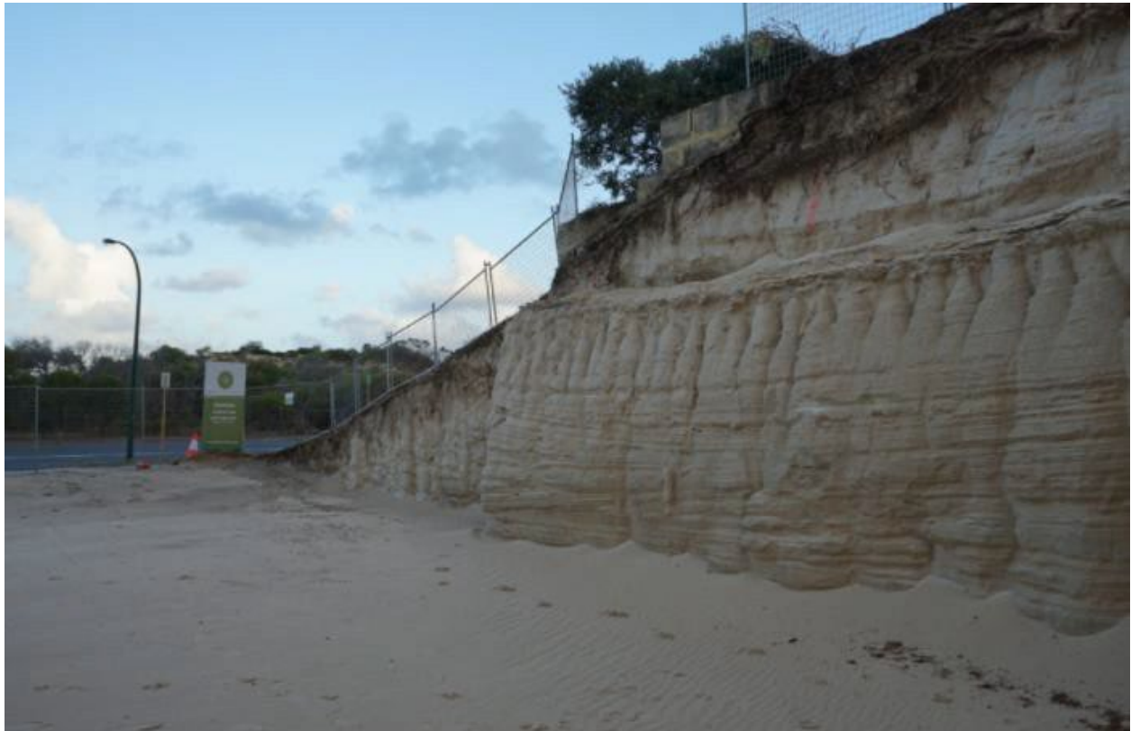
Figure 12. Exposed Permeation Grouting in Sandy Soils
