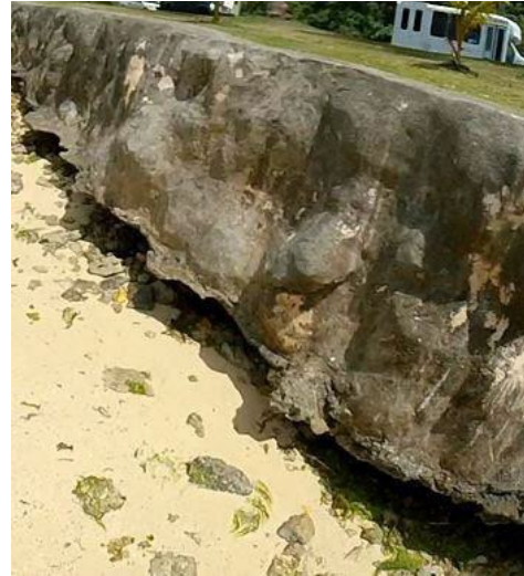
Figure 3. Eastern section of the wall undermined due to erosion
