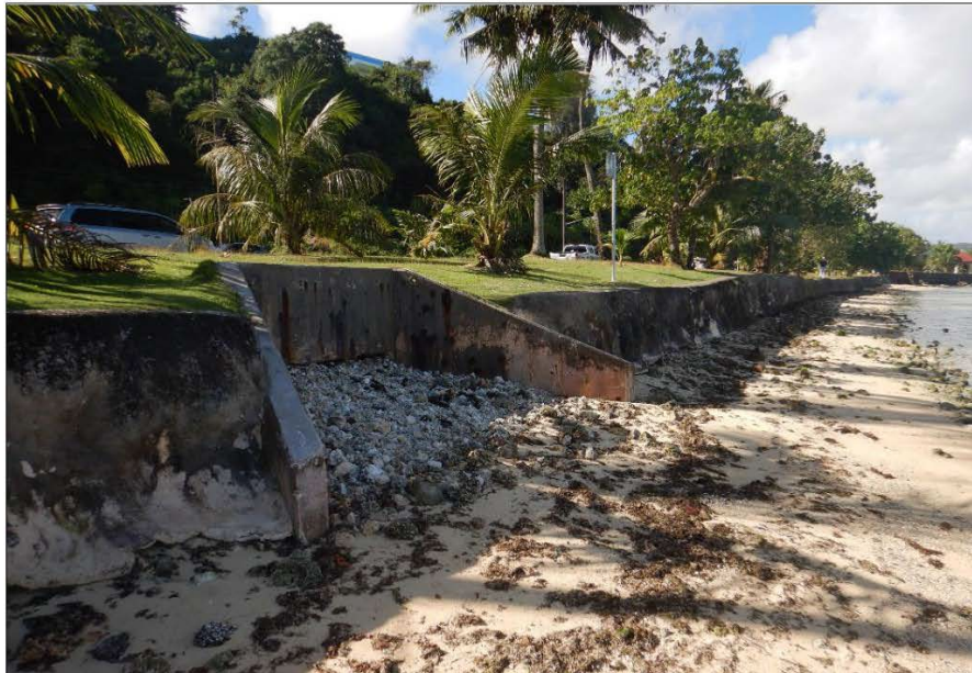
Figure 2. Existing rock seawall along Trinchera Beach.
