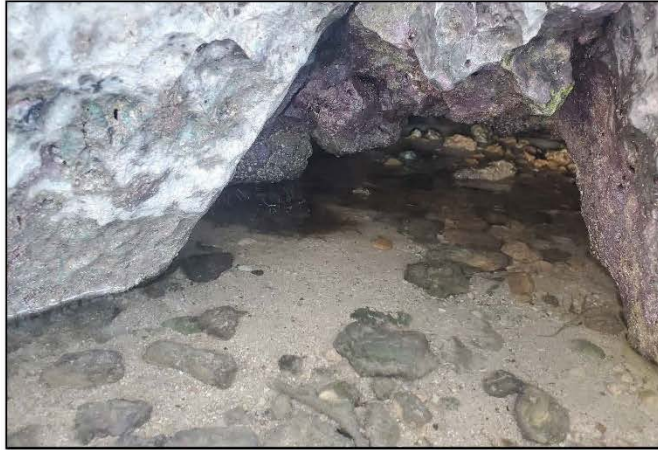
Figure 3: Close up view facing south of the undercut Hagatna Bay seawall (USACE 2022a)
