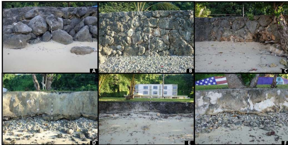
Figure 4. Images of the existing seawall/shoreline from west (A) to east (F) at Hagatna, Guam. The neighboring intertidal substrate consisted primarily of accumulated calcareous sand (A, C, E) with noted regions of aggregated rubble (B) and cobble sized coral skeletons (D and F).
