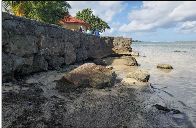
Figure 1: Existing seawall on eastern edge of Veteran's Sunset Beach Park, facing southwest (USACE 2022a). The beach has eroded below the rocks and concrete skirt, causing the seawall to crack, and undermining its structural integrity.
