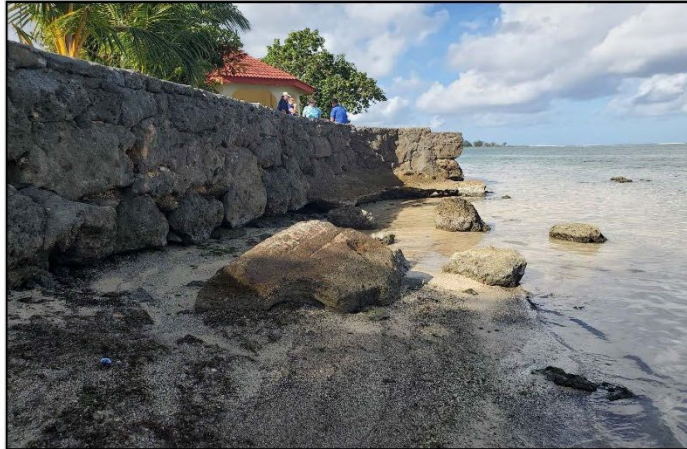
Figure 1: Existing seawall on eastern edge of Veteran's Sunset Beach Park, facing southwest (USACE 2022a). The beach has eroded below the rocks and concrete skirt, causing the seawall to crack, and undermining its structural integrity.
