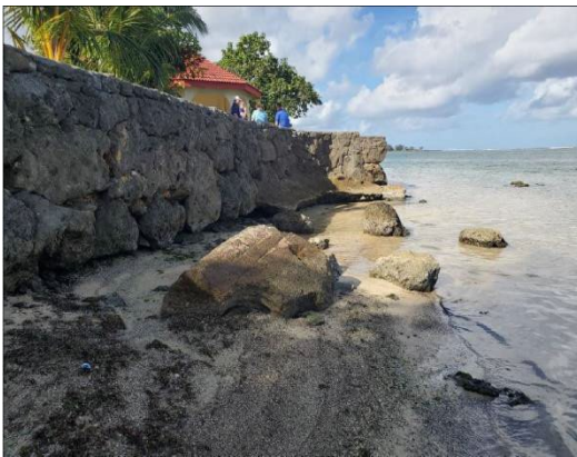
Figure 4. Undermining of the structure around the park pavilion
