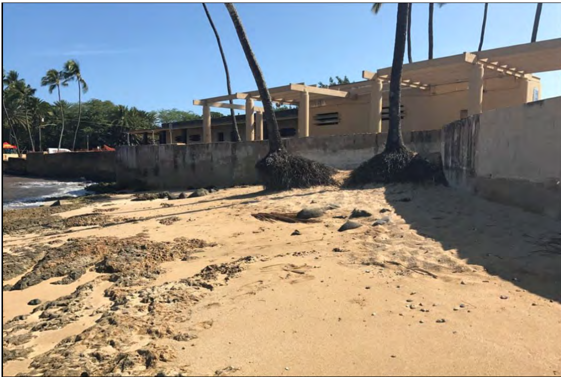
Figure 3. Beach in front of seawall and comfort station. Note exposed reef rock and root balls. Photo from 2017 (Sea Engineering, 2019)
