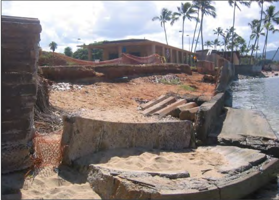
Figure 2-17 Damaged north end of wall (2008)
