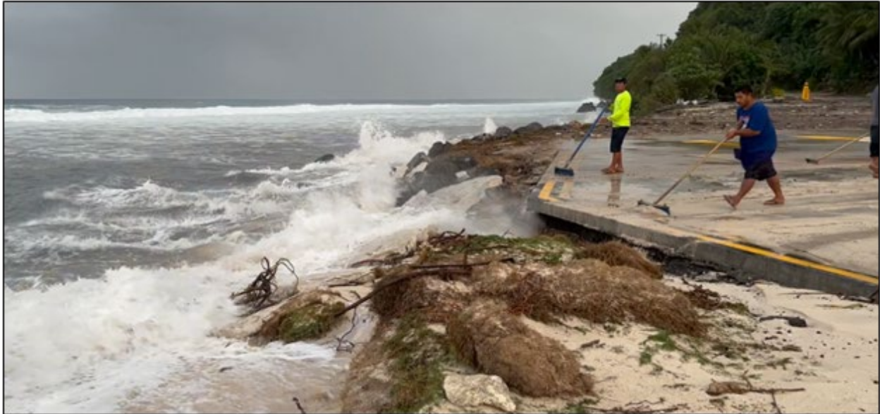
Figure 4: Photos of erosion and damage to runway following extratropical storm event during king tides (photo taken July 14, 2022)
