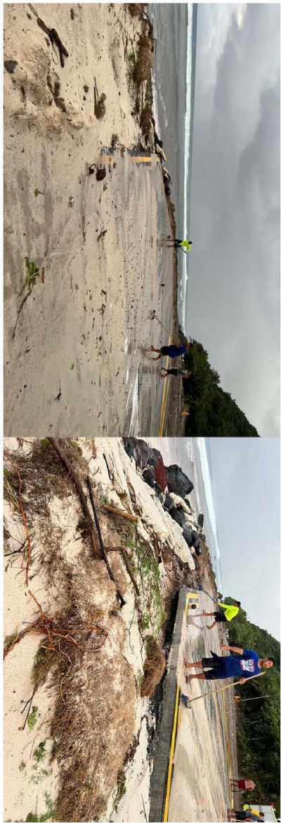
Figure 5: Erosion at New Runway: King tides and large swells combined to impact the newly constructed runway in July of 2022. Photo provided by Corps.
