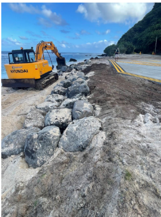
Photo 9. View to the northeast showing heavy machinery working in shoreline protection project area, moving rocks and dirt to repair damage done by king tides and to protect airfield.
