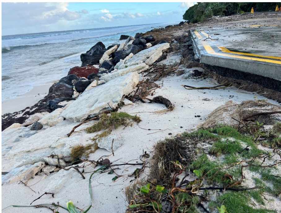
Figure 2. Undermined Runway
