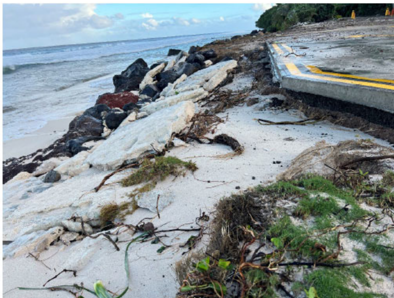
Photo 6. View to the northwest showing undermined runway apron.
