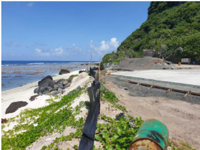
Photo 2. View to the northwest. Silt fence and construction area to top of shoreline bank, batch plant and staging area in the background.
