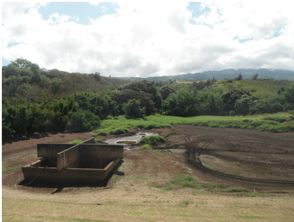
Photo 1-4: Riser structure and saturated conditiosn, Kahana Dam (2017)
