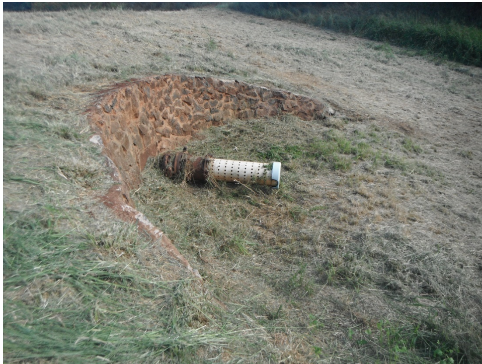
Photo 1-5: Intake for the outlet pipe, Mahinahina Dam
