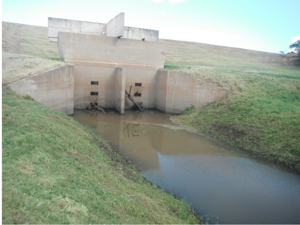
Photo 1-3: Open ports at the riser structure, Honokowai Dam (2017)
