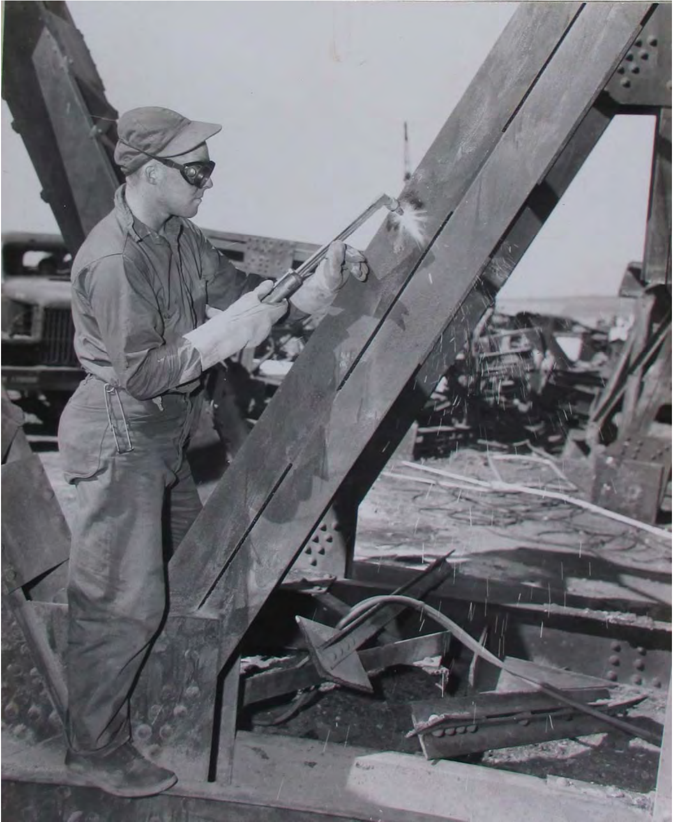
Figure 19 – “Heavy beams are cut with acetylene torches into suitable sizes for shipping at the salvage yard of the Naval Supply Depot of the 14 th Naval District, Pearl Harbor” - 12 February 1945 xix
