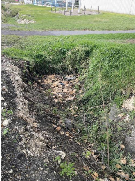
Photo 1. Looking downstream at culvert under pedestrian walkway clogged with leaf litter and debris from recent flow event.
