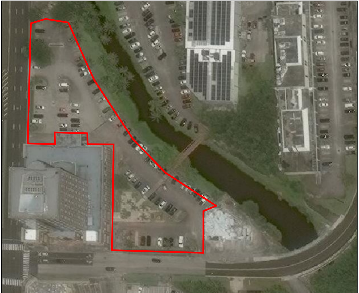
Figure 1. Digital Globe satellite imagery September 19, 2024, with POH-2024-00144 review area in red. The review area consists entirely of an asphalt parking lot. Hagåtña (Agana) River flows through center of image.
