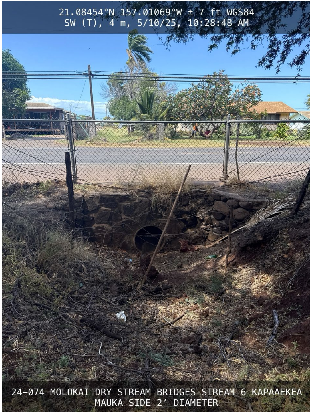
Figure 1- Kapa'akea Stream West looking downstream at Mauna Loa Hwy culvert
