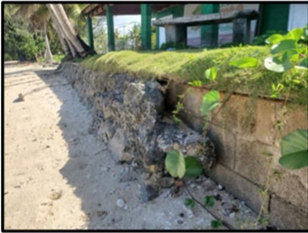
Figures 2 and 3: Erosion and undermining of the existing seawall built to protect the facilities is visible in within the study area. Photos courtesy of The Bureau of Statistics and Plans, Government of Guam
