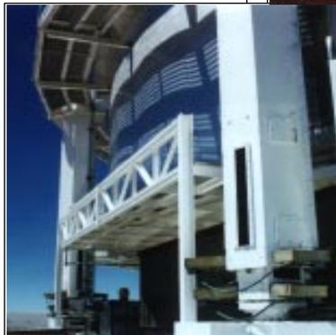
Construction of the \$20 million 3.67-meter Advanced Electro-Optical System (AEOS) telescope at the U.S. Air Force Space Surveillance Complex on the island of Maui is approximately 80-percent complete as it reaches another milestone with installation of the uniquely retracting dome. This 'out-of-the-way' design uses eight 'giant' hydraulic cylinders to move the dome to a position below the base of the telescope and eliminates the vibration associated with
