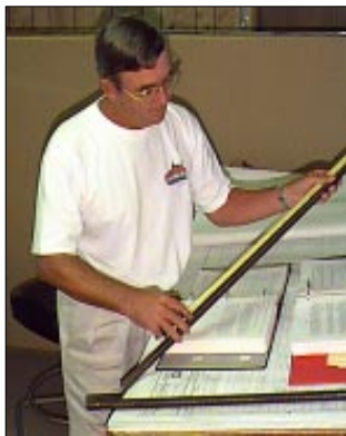
HED construction representative Marty Olson measures pin bolts submitted by the contractor prior to installation. —HED Kwajalein Project Office photo.
