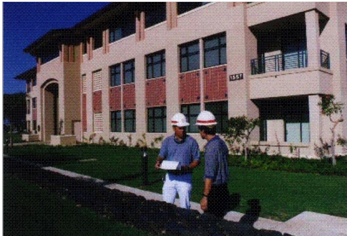
Project engineer Gerald Young, right, and construction representative Randall Chung, HED Fort Shafter Resident Office, inspect the interior and exterior work at the new headquarters building for the IX Regional Support Command, Army Reserve Center at Fort Shafter.
