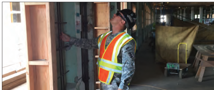
After tearing out the interior plumbing, electrical, and drywall inside a Schofield Barracks Quad building, contractors noticed concrete beams had eroded to a point that compromised the structural integrity of the building. (Above) 1st Lt. David Karwick inspects plumbing lines and amended beams inside a Quad B building. Courtesy photo
