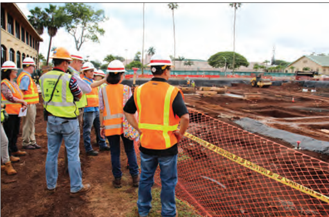
Director of Military Programs Senior Executive Lloyd Caldwell (center), listens as project managers for the Behavioral/Dental Clinic construction project talk about the project progress.
