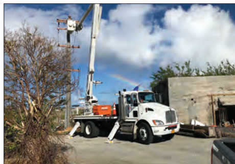
Honolulu District's deployed Power and Planning Response teams working together with Federal Emergency Management Agency (FEMA) installed 160 temporary power generators on Saipan. (Above) The final electrical power re-connection is made to Saipan Airport. Photo by Maj. Brett Fuller
