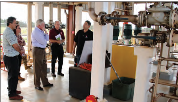
U.S. Army Corps of Engineers Director of Military Programs Senior Executive Lloyd Caldwell (center left) listens as Darin Aihara (right), chief of the Wheeler Army Airfield Resident Office explains the construction timeline for the aviation fuel pump station, which was a part of the 25th Infantry Division Combat Aviation Brigade Phase 1 construction project.
