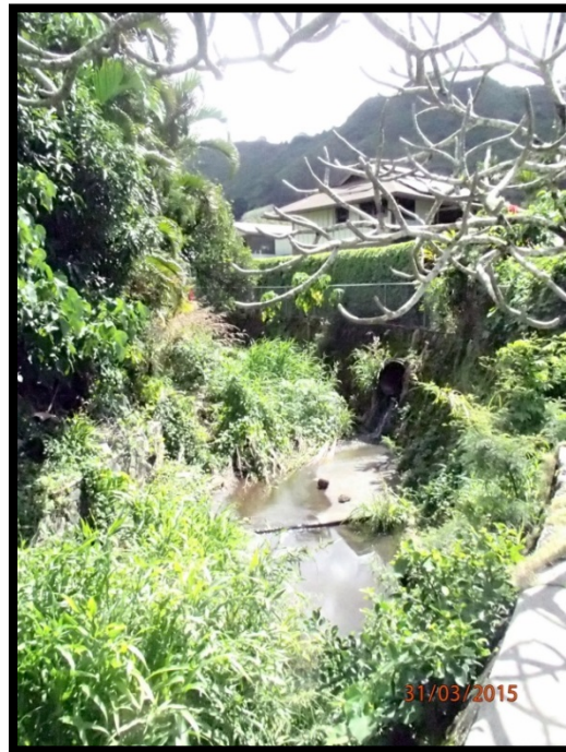
Figure 20: Looking upstream on Woodlawn Ditch from end of Kahiwa Place. Channelized section begins here. (G. Higashi, DAR photo)
