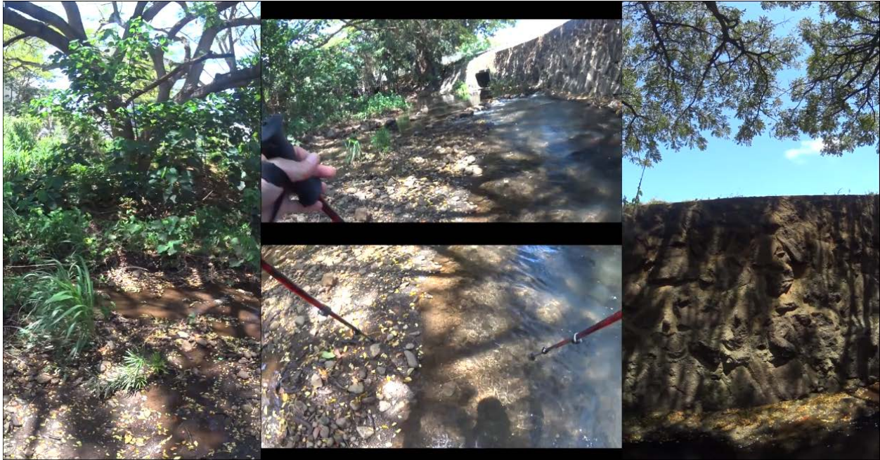
Figure 8: Immediately below the Kanewai Field Intake Site. The large box culvert in upper center image is a reference to the site location.
