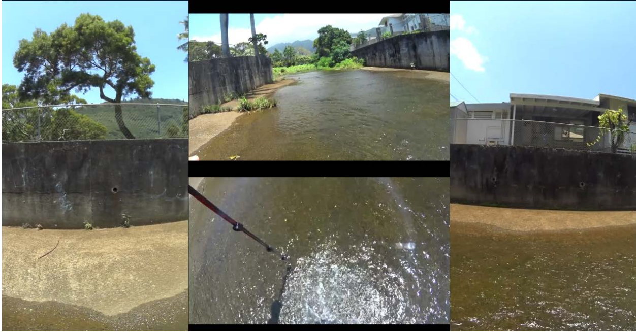
Figure 12: Downstream of Debris Catchment site. Note that the stream is fully channelized here.
