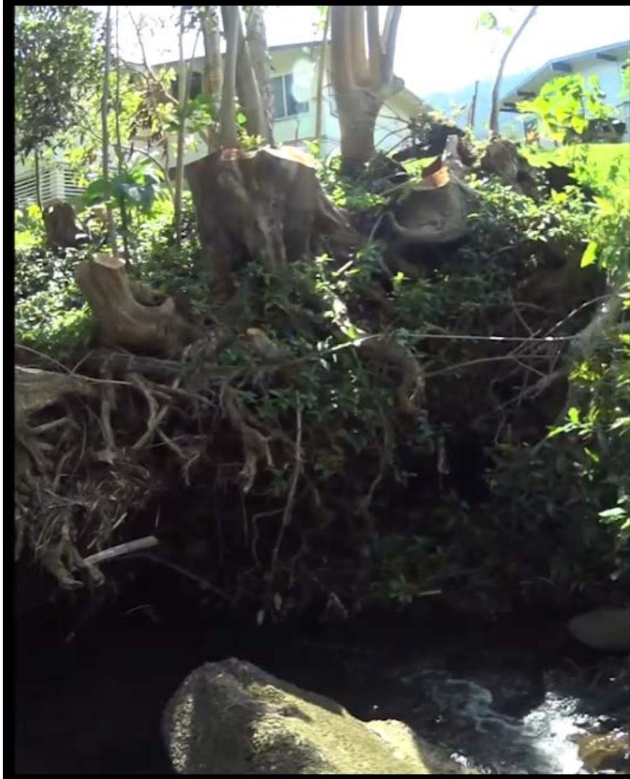
Figure 97: Extreme streambank angle ( >90^\circ , or undercut).
