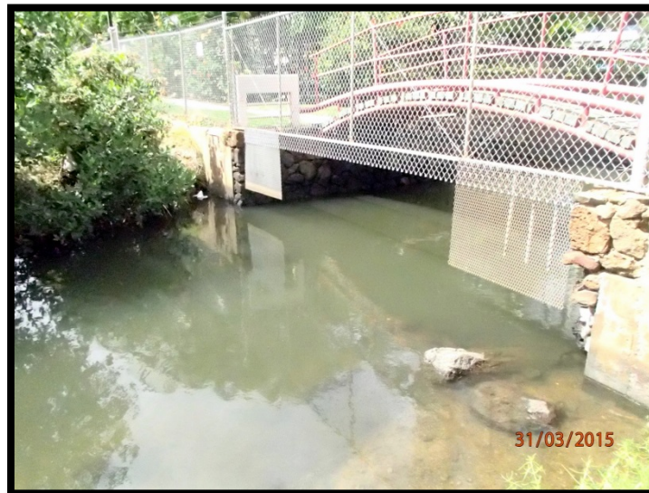
Figure 43: The boundary fence for the Marco Polo Apartments on Hausten Ditch.
