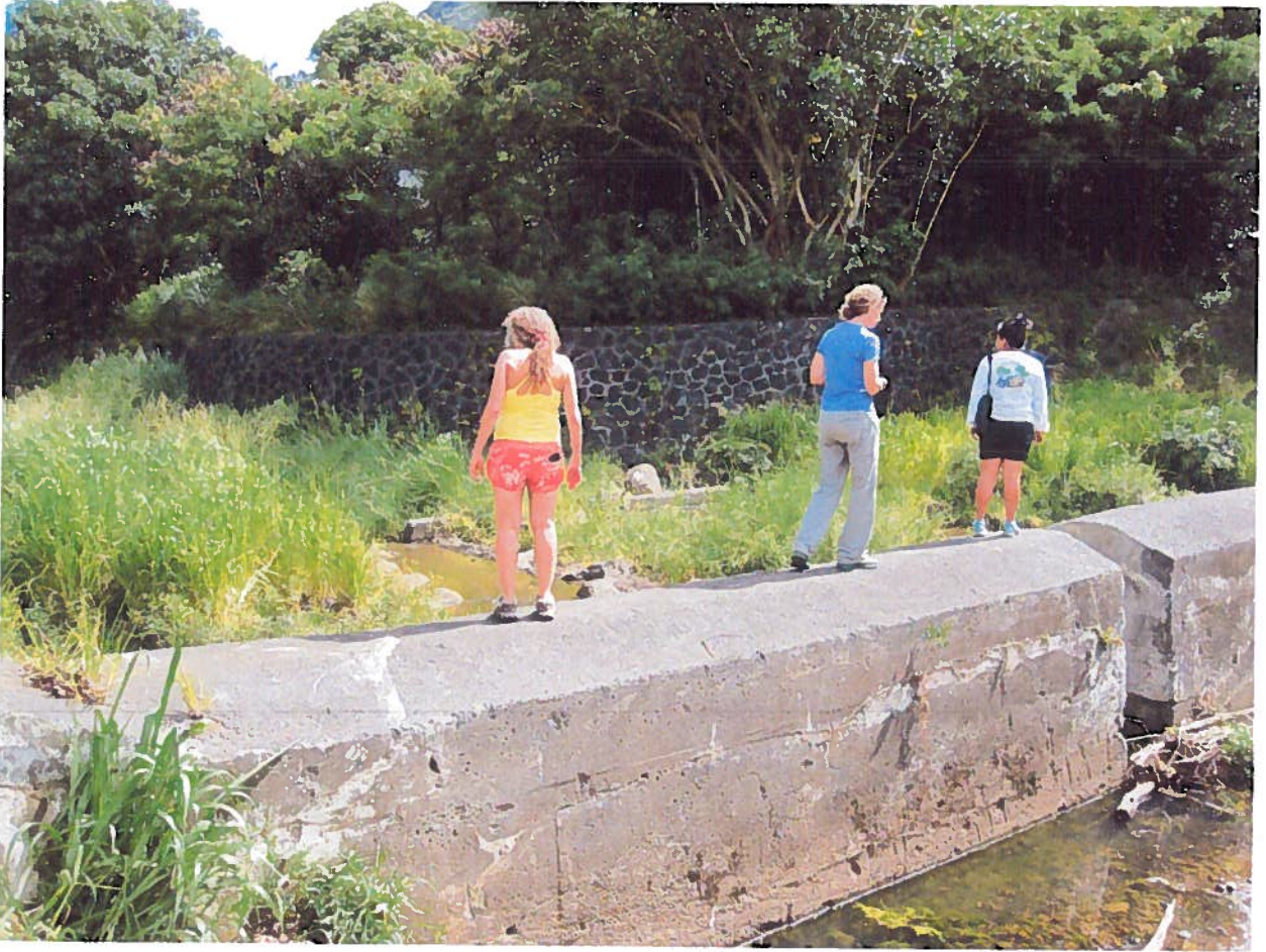
Figure B-5. Examples of Maintenance Dredging in Detention Basin Pool Area – Culvert.
