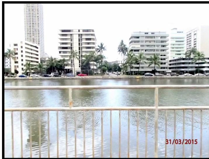
Figure 40: Looking downstream toward the Ala Wai Canal from the first pedestrian bridge over Hausten Ditch.
