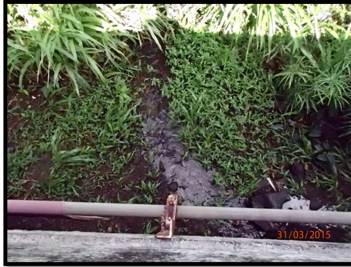
Figure 19: View straight down from East Manoa Road Bridge into Woodlawn Ditch. (G. Higashi, DAR photo)
