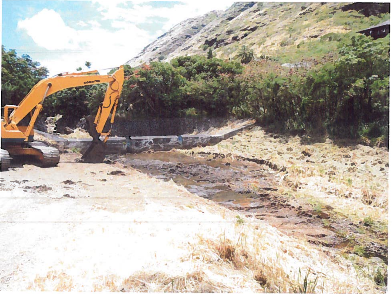
Figure B-4. Examples of Maintenance Dredging in Detention Basin Pool Area – Backhoe removing debris from stream.
