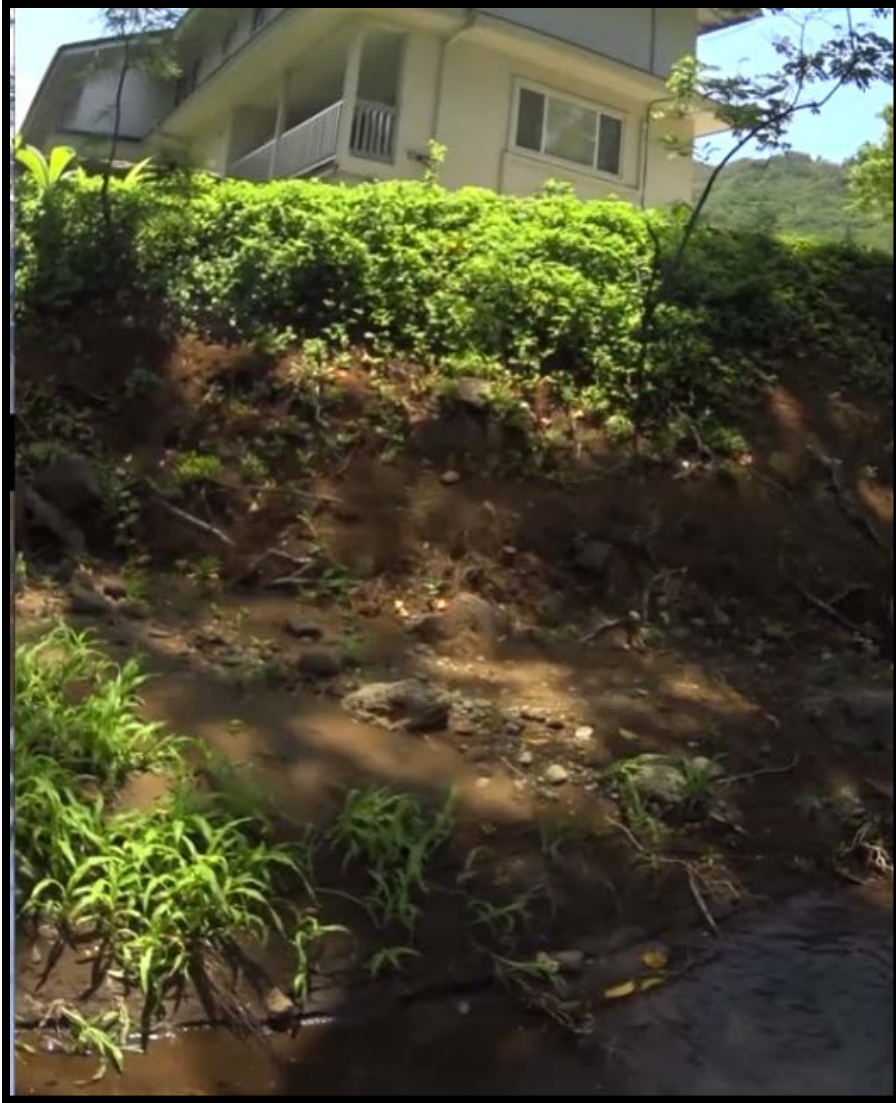
Figure 99: Poor and Marginal streambank surface protection. Here the bank is transitioning from an area of poor surface protection (right) to marginal surface protection (left). Note the high potential for surface erosion at this location.
