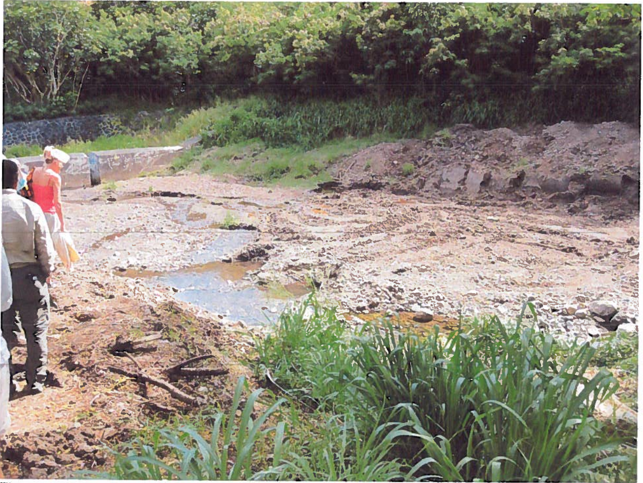
Figure B-2. Examples of Maintenance Dredging in Detention Basin Pool Area – Exposed soil and altered stream.
