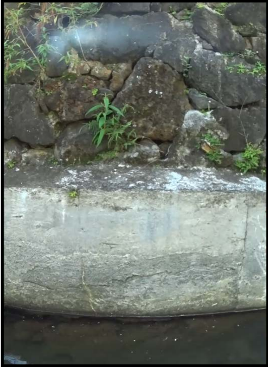
Figure 96: High streambank angle (near 90°).
