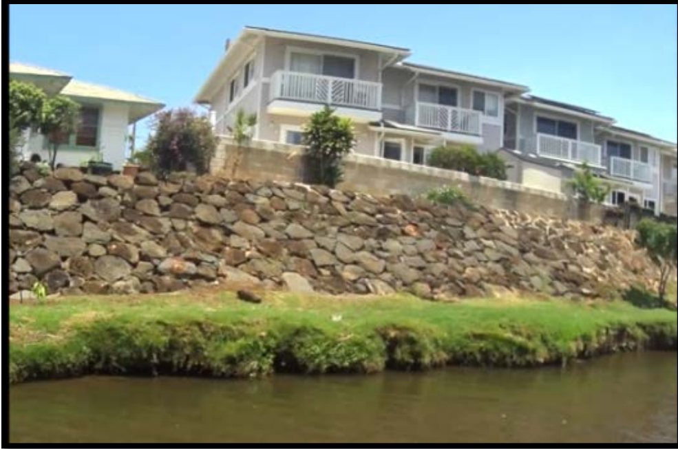
Figure 94: Streambank Height class for greater than 18 ft. This image highlights the scoring when a flood wall is close to the streambank. Where the wall is close, the bank height equals the height of the wall. If the wall had been set further back, then height would equal the first bench in the front.
