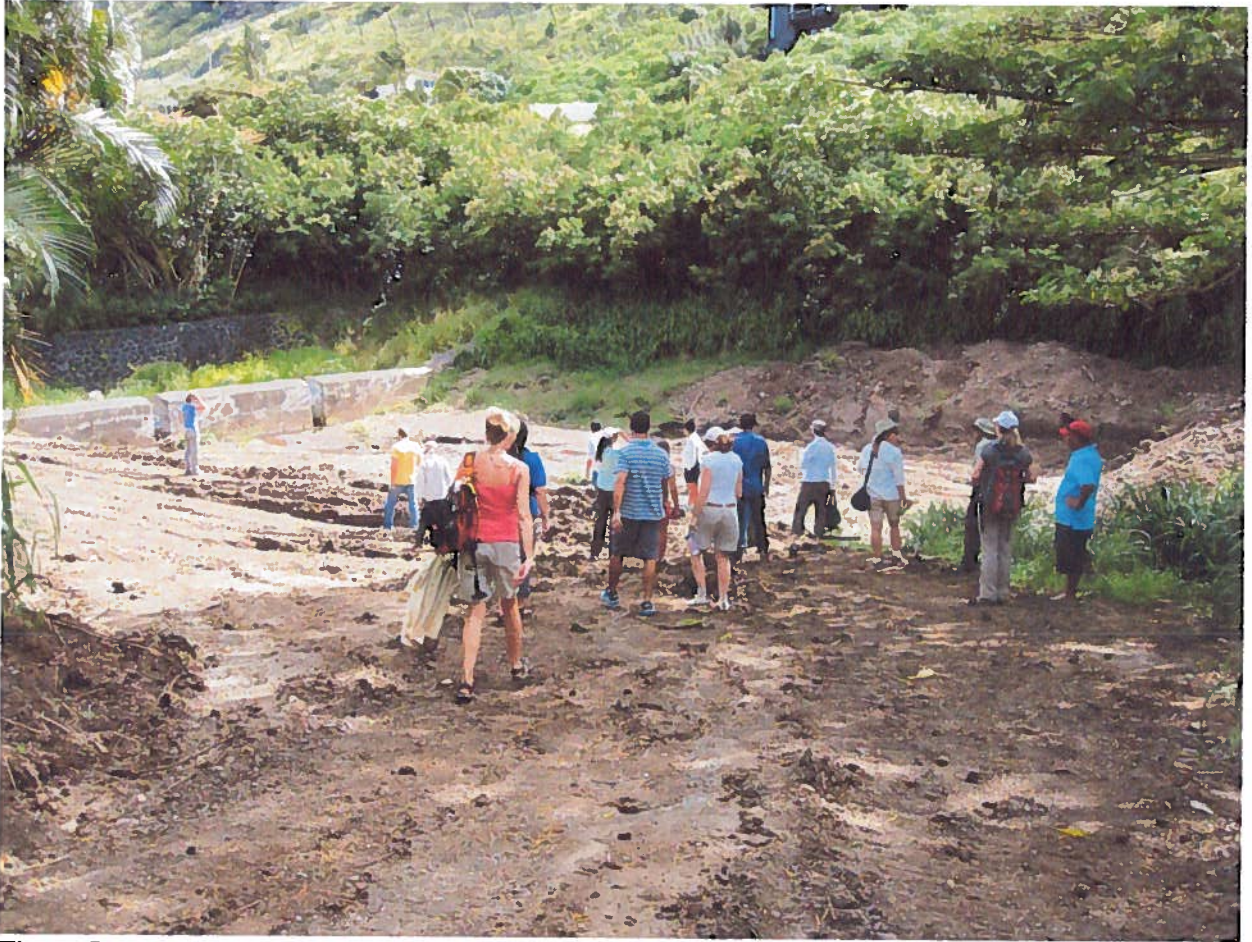
Figure B-1. Examples of Maintenance Dredging in Detention Basin Pool Area – Vegetation and debris removed and soil exposed by bulldozer.
