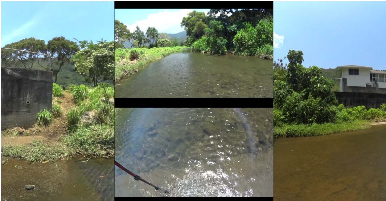
Figure 13: At the end of the channelized section immediately downstream of the Debris Catchment site.
