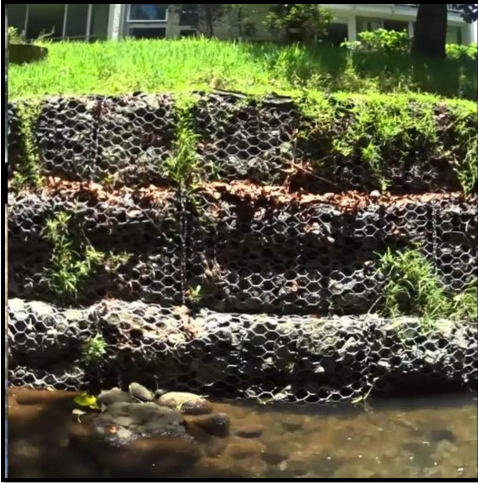
Figure 104: Low Potential for Bank Erosion. Bank Angle is just under vertical and the Bank Surface Protection is highly protected due to gabion baskets. There is no riparian diversity which means no root structure to hold together the rocks, but this has been functionally replaced by the braided wire fence.
