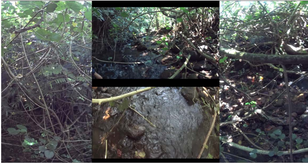
Figure 28: Lower end of Waiakeakua Debris Basin. Note that much of the area is overgrown by Hau trees.
