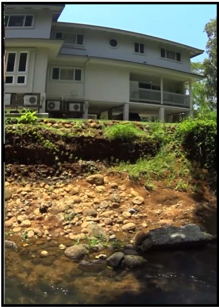
Figure 100: Poor Riparian Zone Condition. No trees, shrubs or tall grasses to provide shading.
