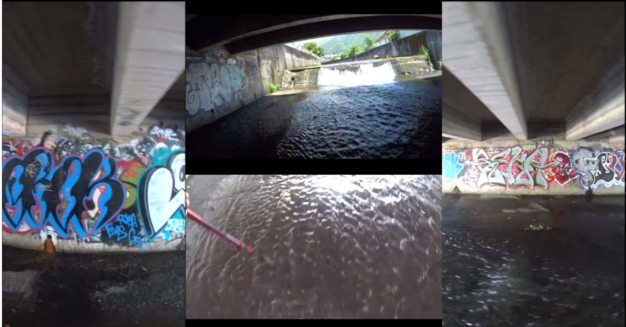
Figure 49: Drop in the channelized segment of Manoa Stream.
