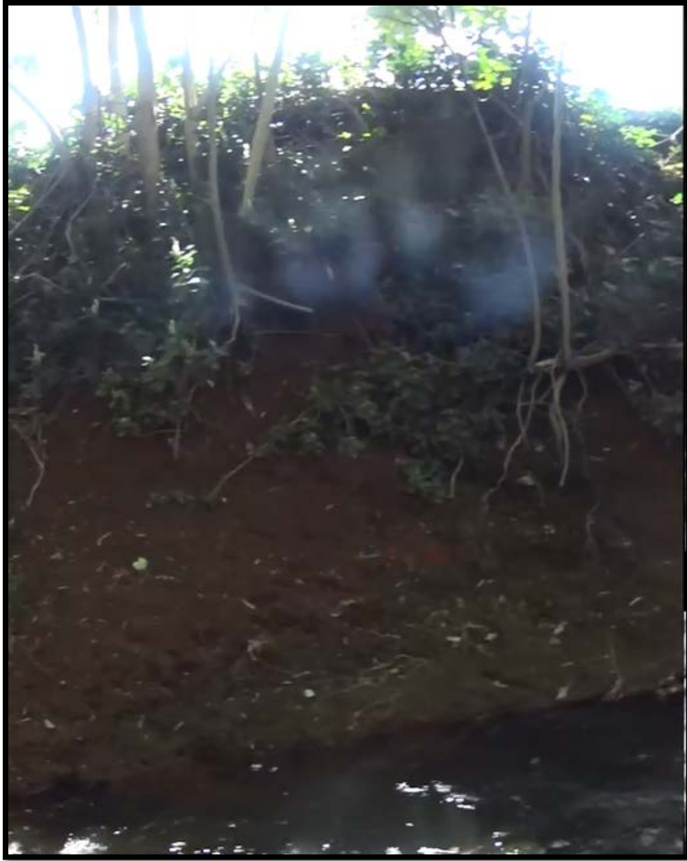
Figure 106: High potential for Bank Erosion. The bank shows an almost undercut bank angle with marginal surface protection due to limited vegetation on the top part of bank and poor riparian diversity due to the complete lack of roots. Bank erosion is likely during high water events.
