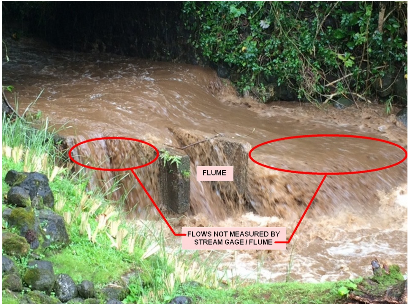
Figure 2 – Waiakeakua Stream Gage / Flume During Storm Conditions
