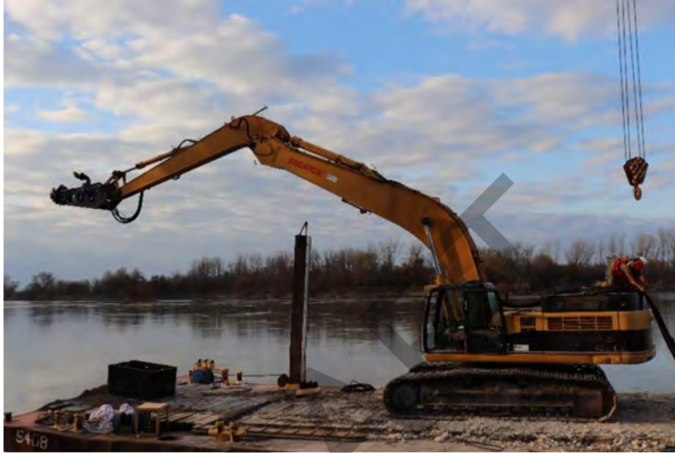
Figure 10 Example Excavator Staged atop Barge
