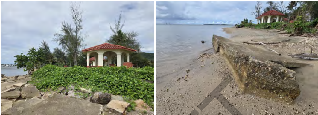
Figure 8 Example Concrete and Other Debris Along Shoreline
