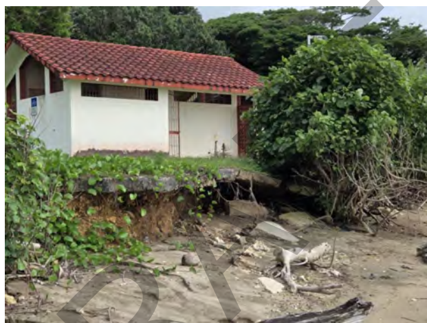
Figure 5 Erosion at south end of Nimitz Beach as of Sep 2025. Escarpment is 4 to 6 feet tall. (USACE 2025)
