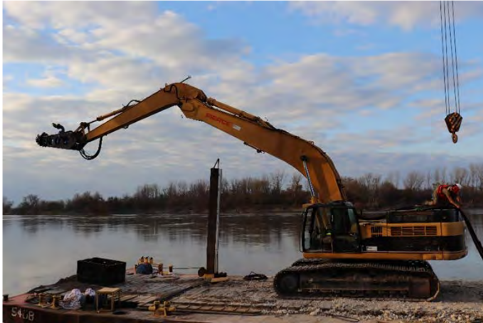
Figure 4 Example Excavator Staged atop Barge
