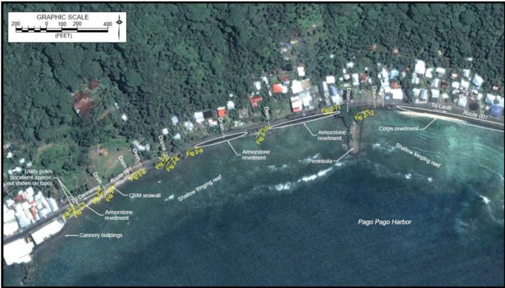
ATTACHMENT 1 Project Location Map Route 1: Proposed Amorstone Revetment Corps File No. POH-2015-00249 (Atuu to Laulii Shoreline Revetment Protection Project)
