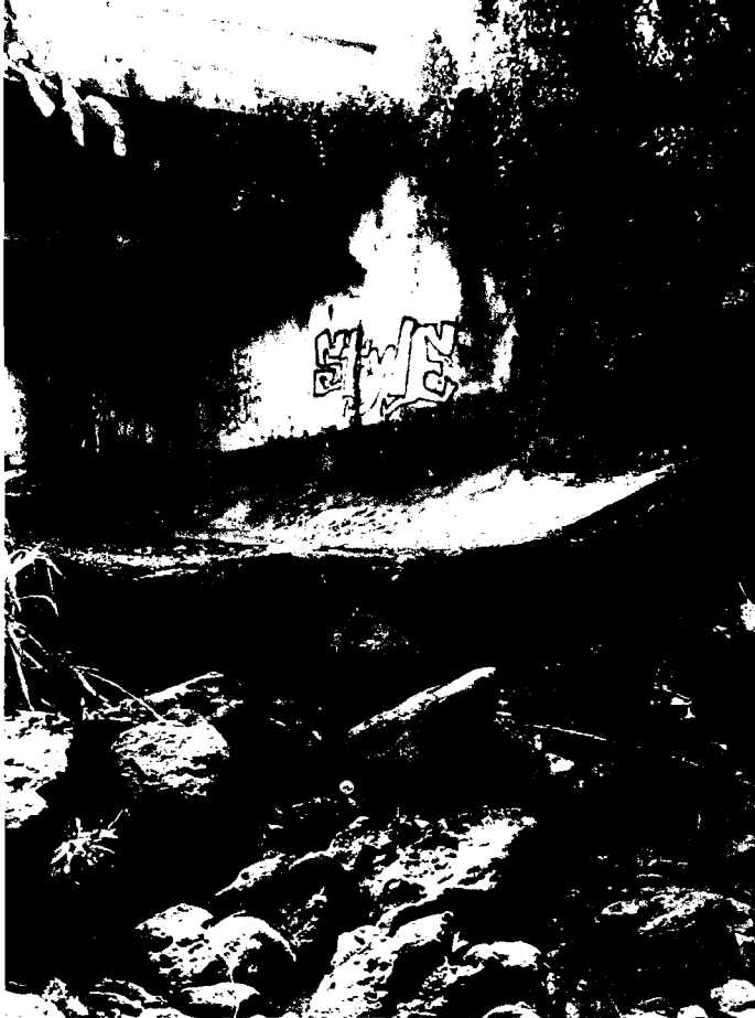
5. Looking upstream at top of project site. Note eroding condition of invert and undercut toe where high velocity stream water discharges.
